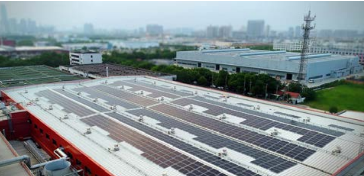
Kunshan Integrated Site in China
