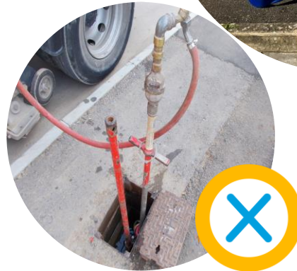
Thames Water authorised standpipes (above) and an illegal connection (left)
