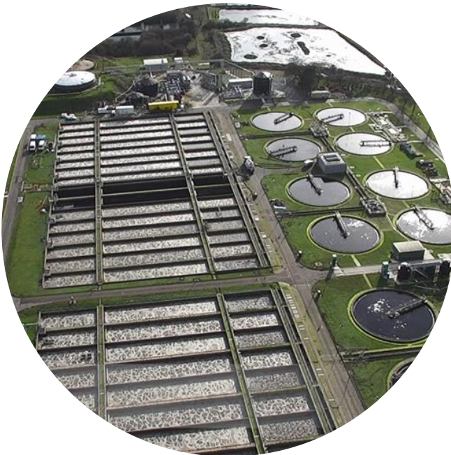
Aeration lanes and settlement tanks used for conventional activated sludge process.
