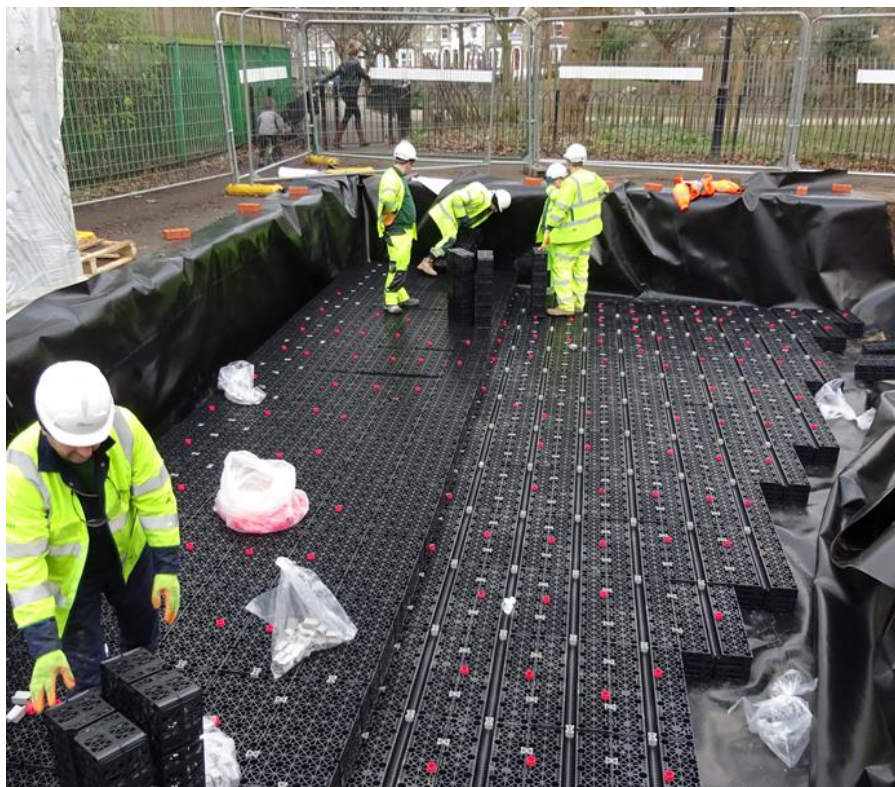
Installing sustainable drainage in west London.
