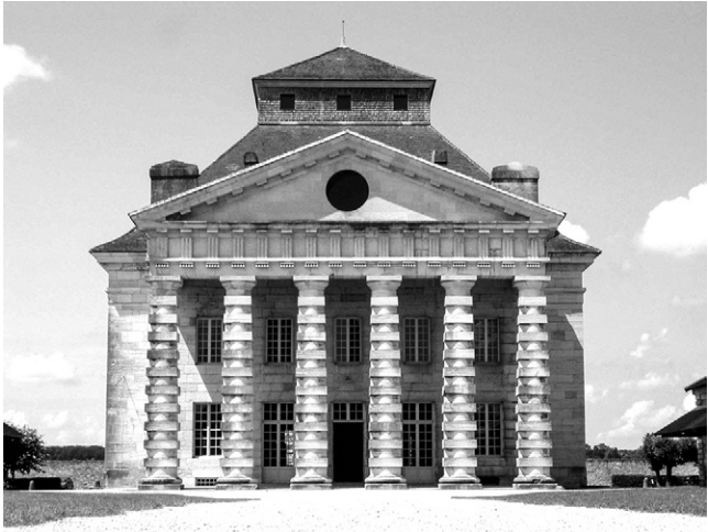
home of the overseer ( temple du surveillance ), designed by Claude-Nicholas Ledoux, ca. 1780. Current view.
