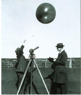
This image shows early testing of hydrogen-filled balloons for radiosonde measurements. The theodolite in the image was used to track the balloon to the limit of visibility.
