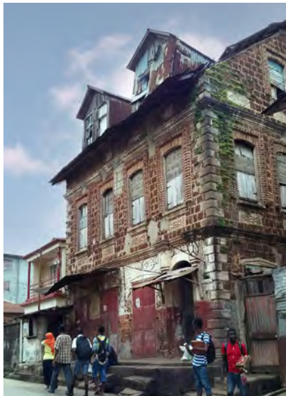
Residential vernacular heritage includes Krio board houses as well as masonry houses constructed with local laterite.
