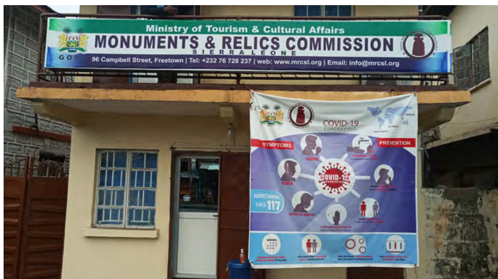
Current headquarters of Monuments and Relics Commission in Freetown.
