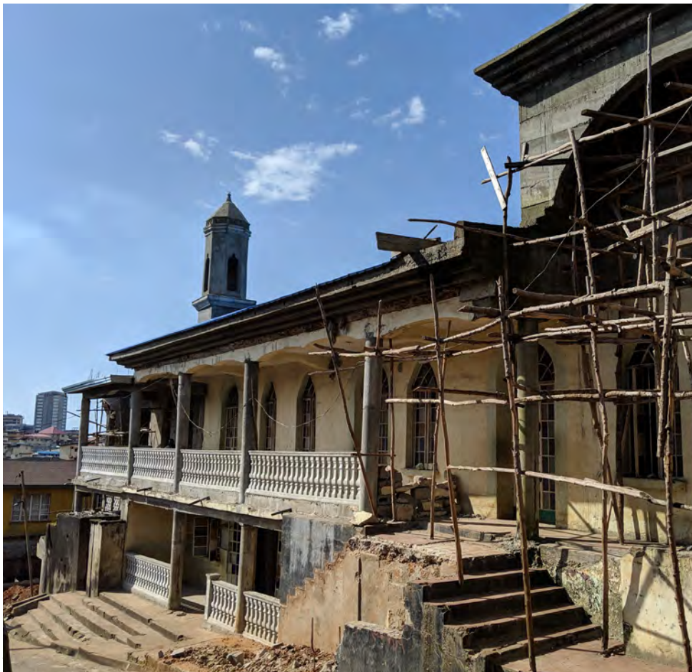
Jamaat ul Salaam Mosque is undergoing renovation and expansion.
