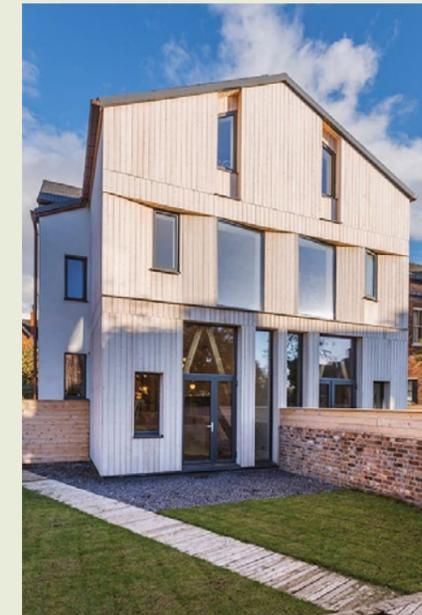
use of biocides and resisting rot and ultraviolet degradation for 30 years. Windows are angled towards the sun, within the insulation layer, to maximise passive solar gain. Each layer of the walls, roof and floors is highly breathable to allow drying both inside and out should moisture get in in the future.
