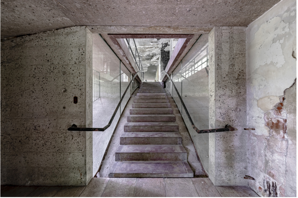
Lower view of the Casa sobre el Arroyo's stairwell before restoration.
