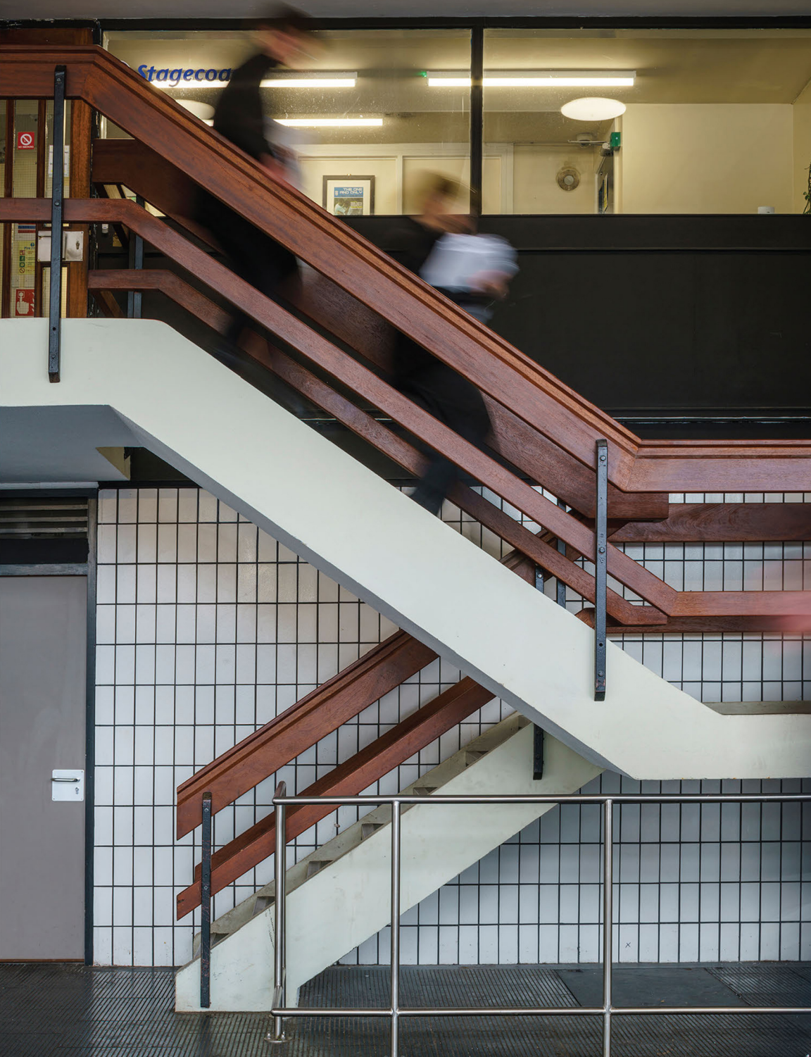
Stair after restoration.
