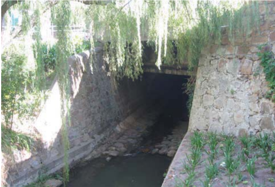
The headwall of the original bridge built at Westerford in 1814, which crossed the stream at right angles thereby necessitating a kink in Main Road, is still visible alongside the modern bridge at the start of the Liesbeek Trail. (Photo: Cate Brown)
