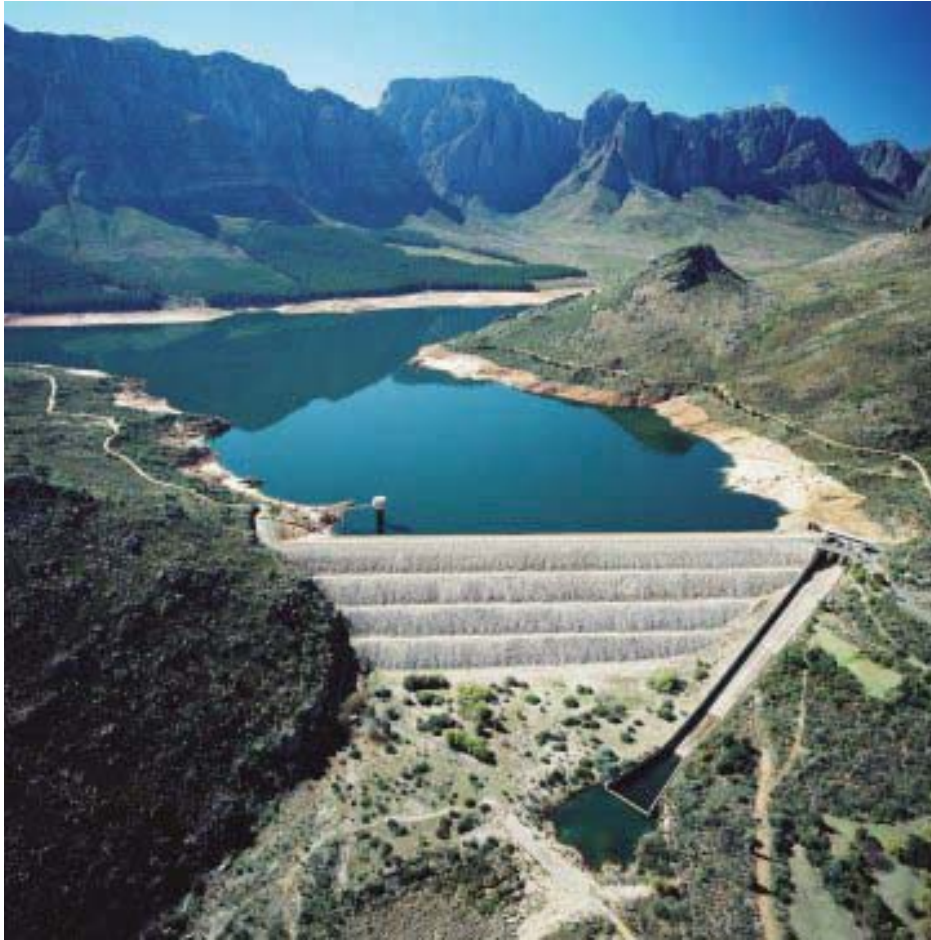
Wemmershoek dam wall (Photo: City of Cape Town Archives)
