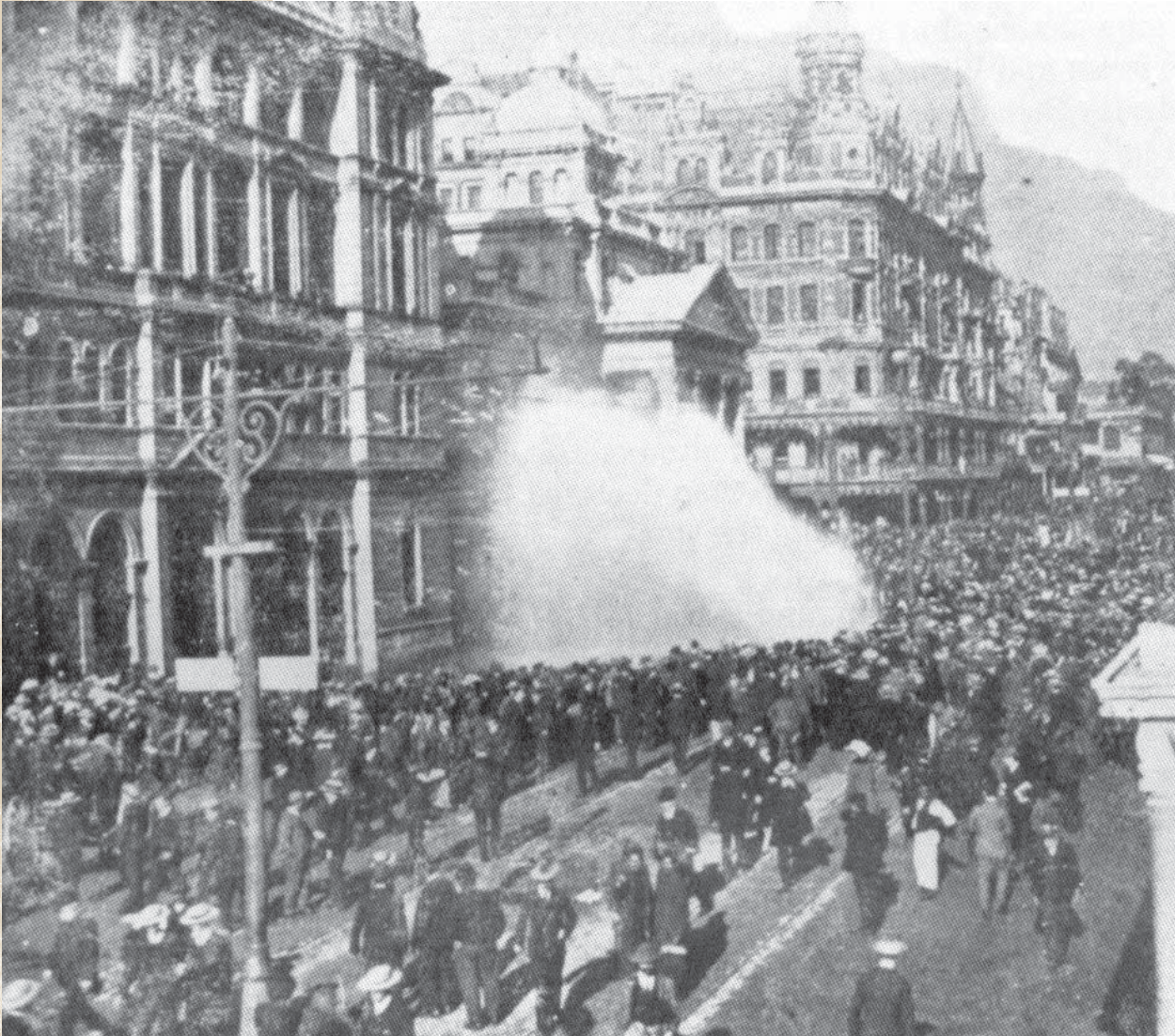
Burst water main after the gas explosion in Adderley Street, 1905 (City of Cape Town Archives)
