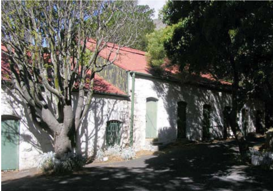
The Platteklip washhouses circa 2003, before their renovation for use as accommodation for hikers on the Hoerikwaggo Trail (Photo: Jenny Day)
