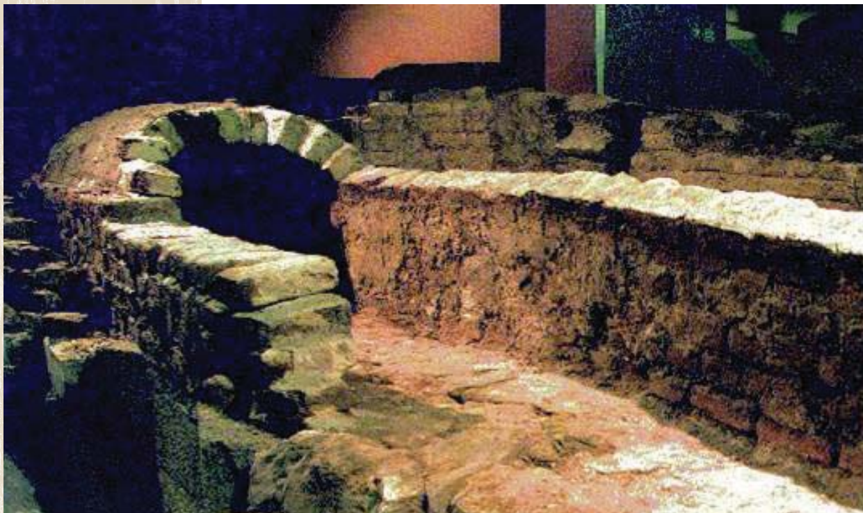
Wagner's Reservoir, "sixteen roods by four and half a rood deep", can be seen today on the lower level of the Golden Acre Shopping Centre, Cape Town (Photo: Tony Murray)
