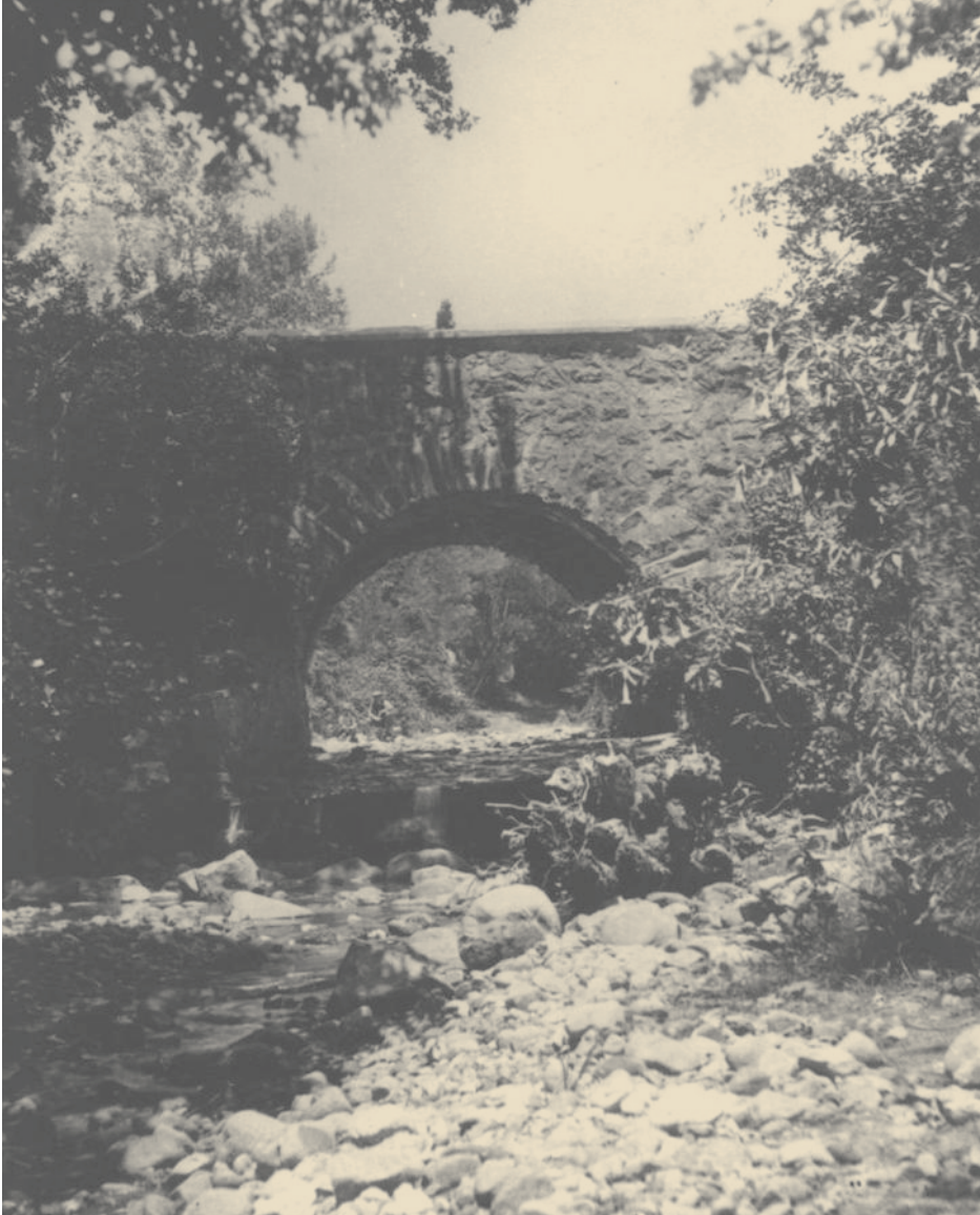
The Westervoort Bridge, named after Westervoort Farm, was built across the Liesbeek in 1814 at the site of the ford that had been in use since 1689 (Western Cape Archives)
