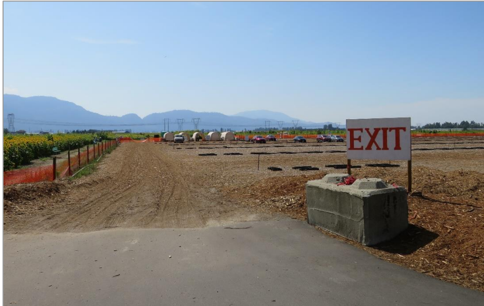
Photo 5 Red cedar hog fuel used to create an in-field parking lot for U-pick operation in the Fraser Valley.
