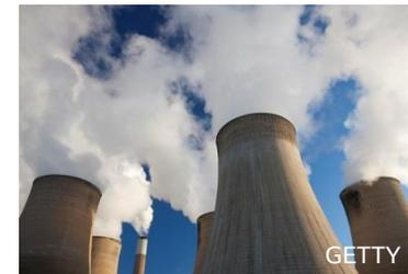
Biomass is burned in power stations to create electricity
