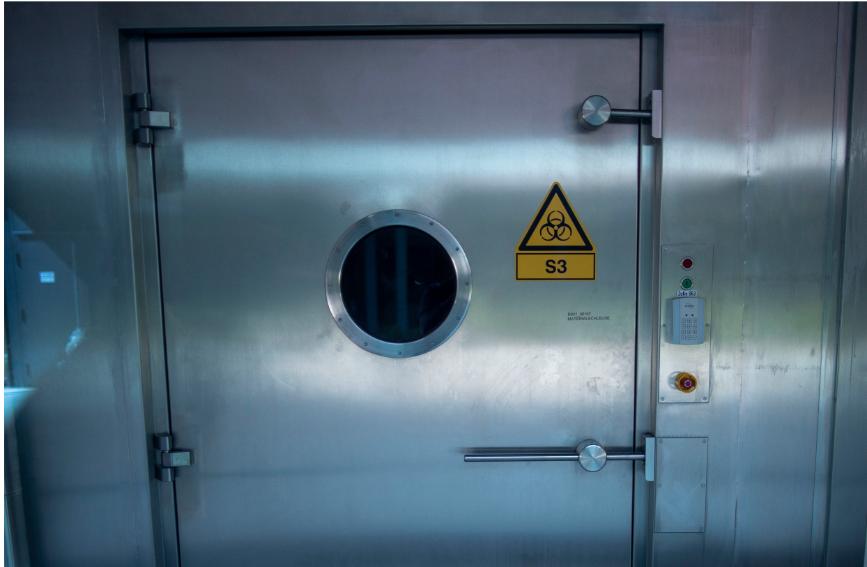
Special airlock doors are seen in front of a security level 3 laboratory in a building of the Friedrich-Loeffler-Institut on the island of Riems, Germany, on July 2, 2020. (Jens Büttner/picture alliance via Getty Images)
