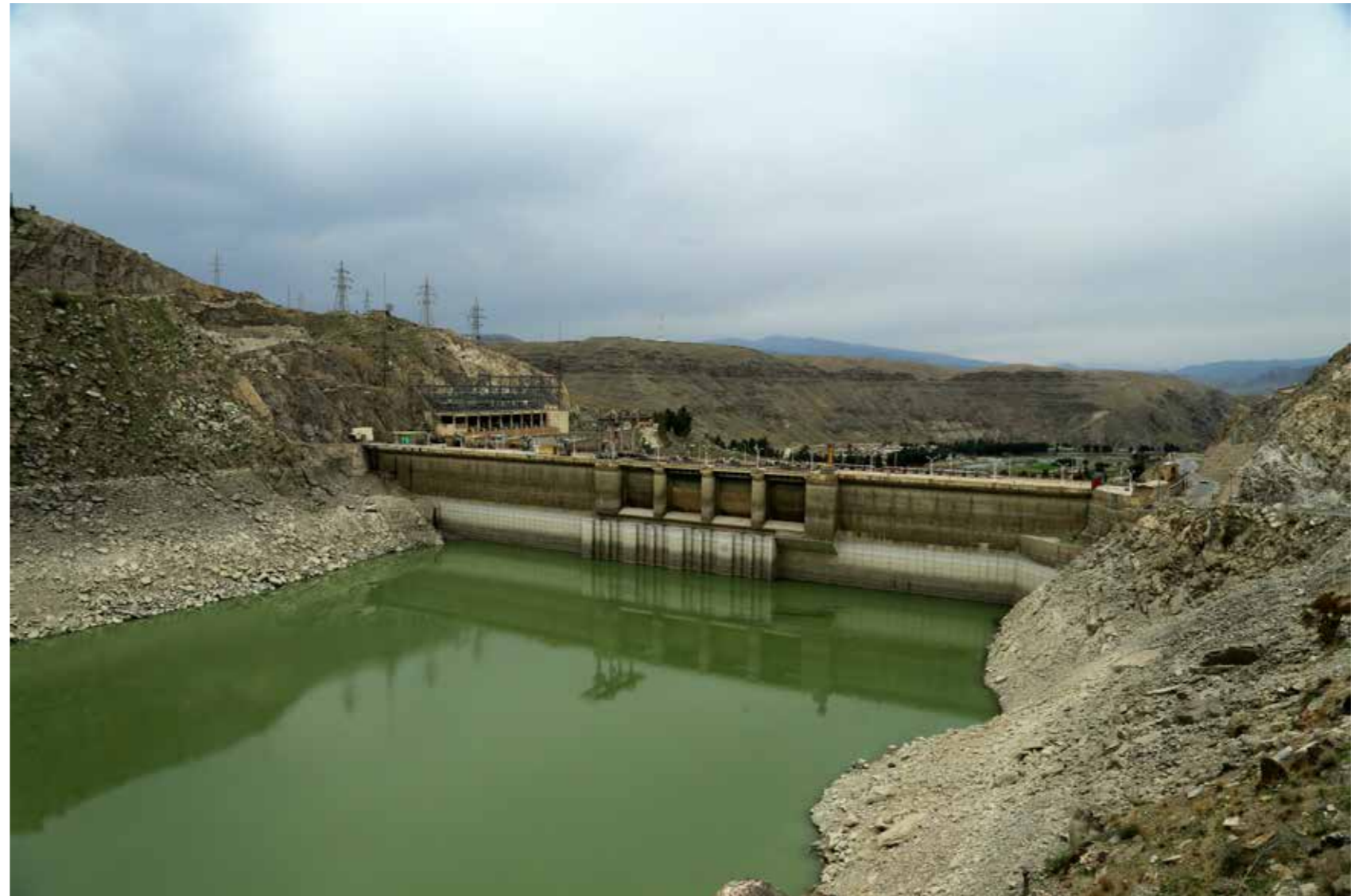
Rehabilitation of the Naghlu Hydropower Plant is progressing well. As part of local development assistance, NHRP intends to provide electricity in areas close to the Naghlu dam. Residents in several villages in two districts close by will benefit from the project.
