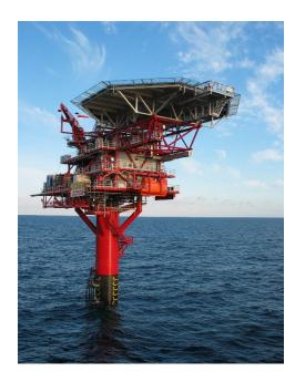
Figure 0-28: Unmanned wellhead platform [20]
