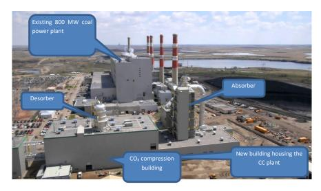
Figure 13. Photo [37] of Saskpower 800 MW<sub>e</sub> Boundary Dam coal-fired power station where one of the four units was retrofitted with amine CC in 2013.
