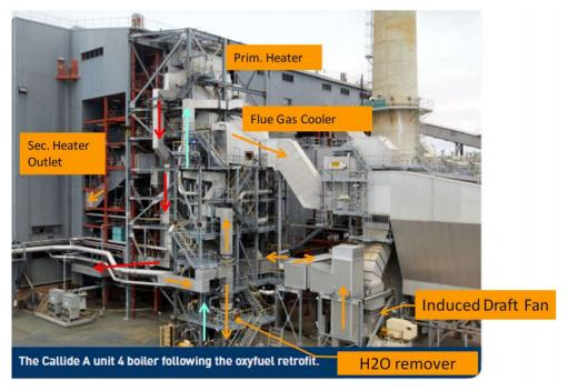
Figure 31 Photo of Callide Oxy-fuel boiler from [11] showing retrofit paths (red) and flue gas flue directions (yellow).
