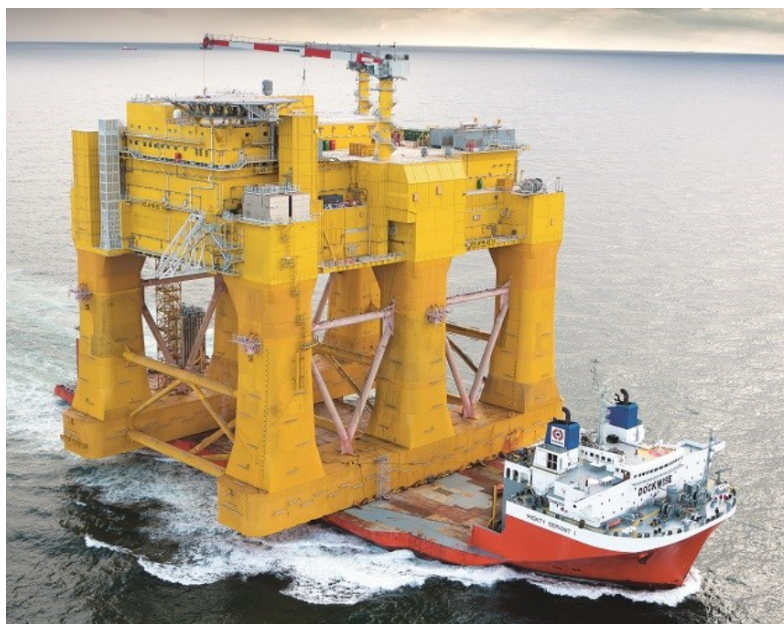
Figur 8-10 Dolwin 2 transformer platformtransport.
