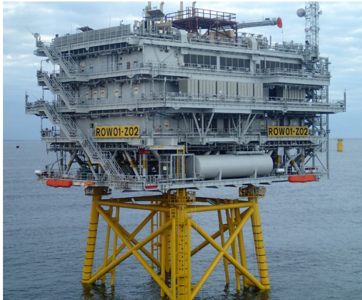
Figur 8-4 Traditionel AC-transformer platform- Ørsted Race Bank Vindmølle Park.
