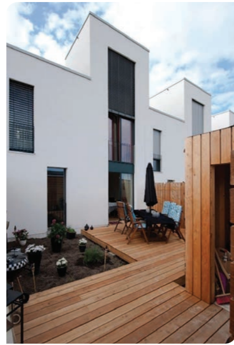
New social housing in Denmark
