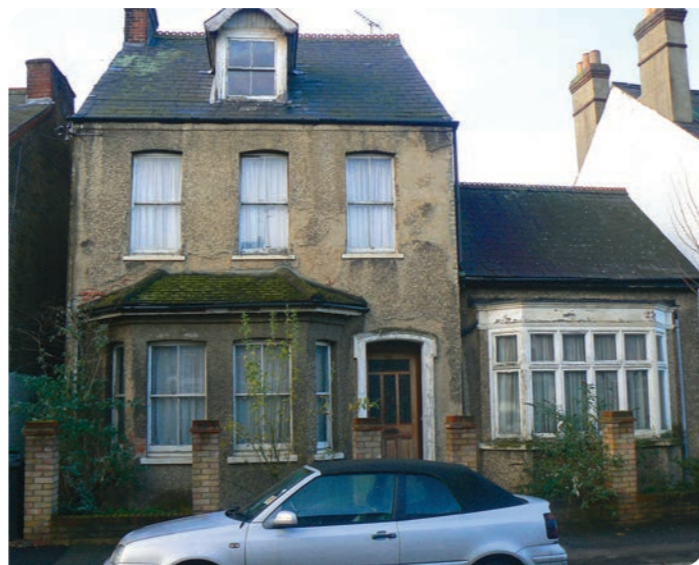
Photos: Older homes are more likely to be in disrepair
