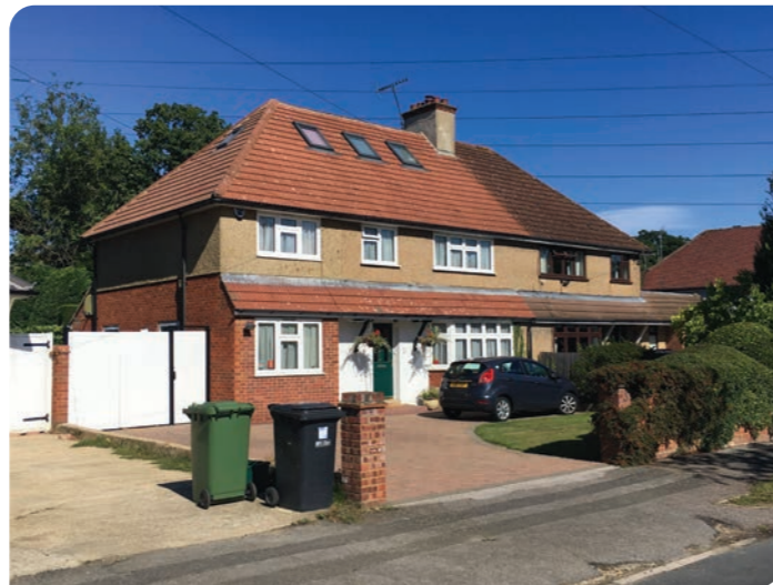
Photo: A modest suburban 1930s semi-detached house, now improved to 5 beds with side, rear and loft extensions
