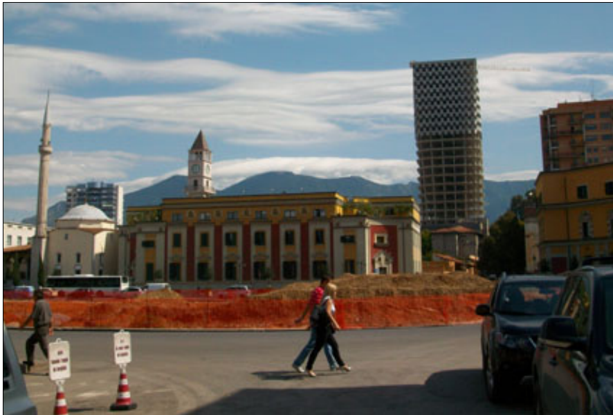
Fig. 15. Part of Skanderbeg Square. From the left: Et'hem Bey mosque, one of the Italian built ministry buildings with the clock tower behind it, and the first of ten new towers which will be built around the square.
