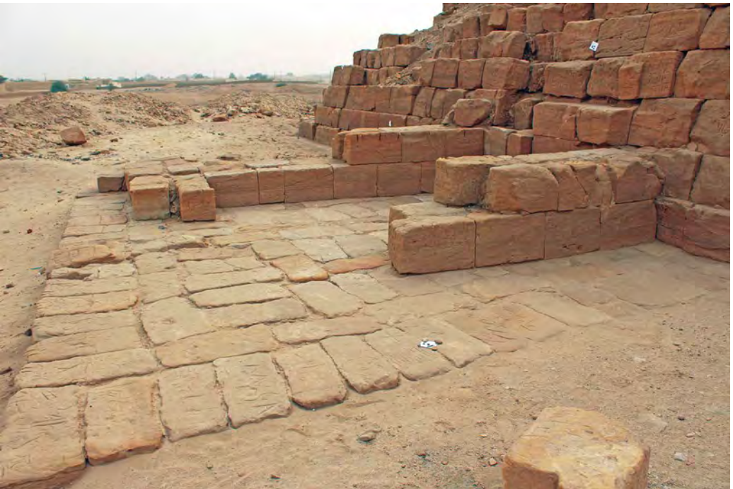
FIGURE C.9. East face, exterior of north chapel wall. Photo: IKAP
