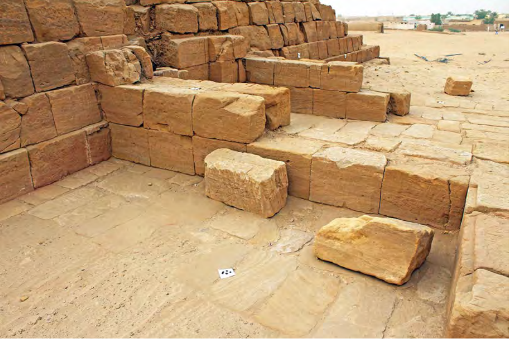
FIGURE C.8. East face, exterior of south chapel wall. Photo: IKAP
