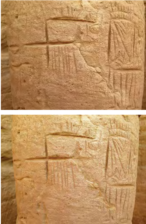
FIGURE 4.5. A cracked graffiti before (top) and after (bottom) fine-grouting with Voidspan.
