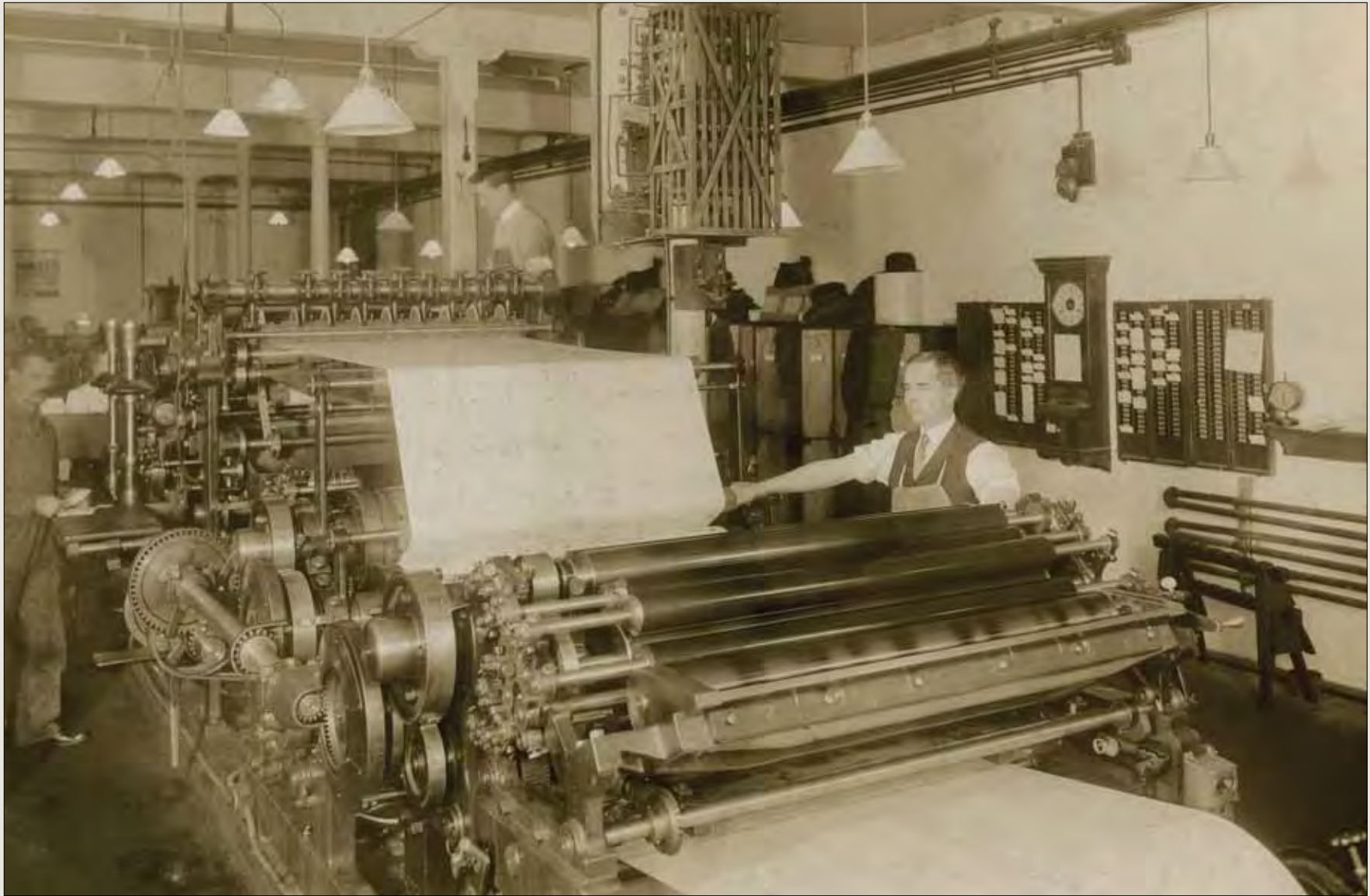
Close-up of the same web press in the old building, about 1900.
