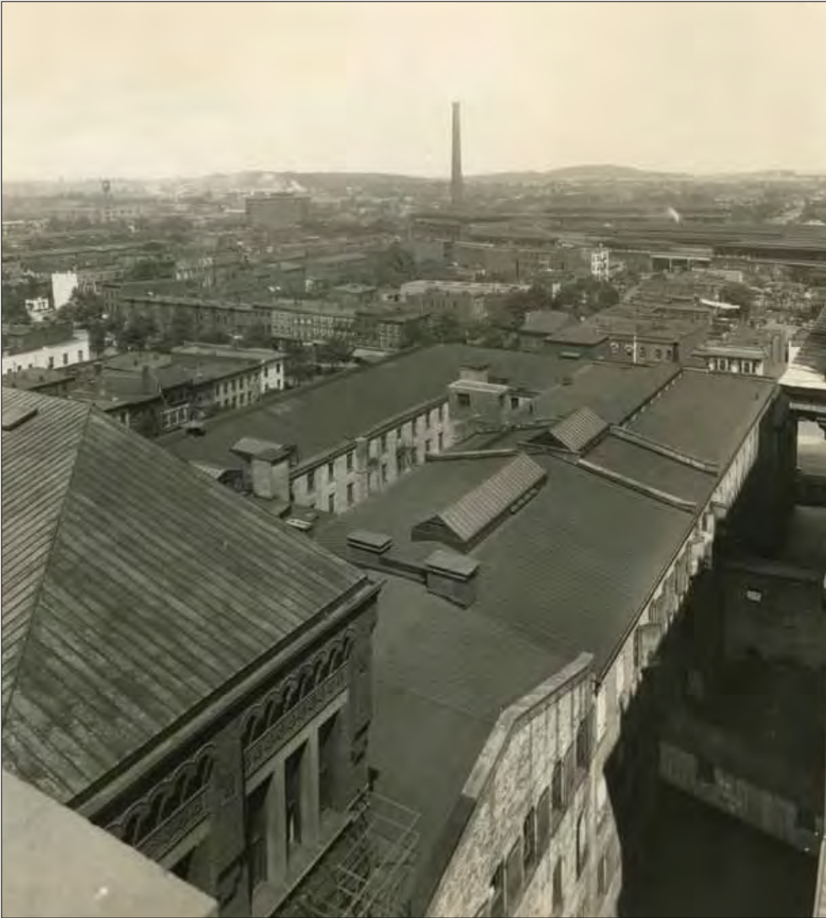
This view from the roof of Building 2 looks over the rooftops of the old building complex, with the tall narrow annex at left. Swampoodle is more densely residential, and the city has grown up all around. The tracks of Union Station are visible in the middle distance.
