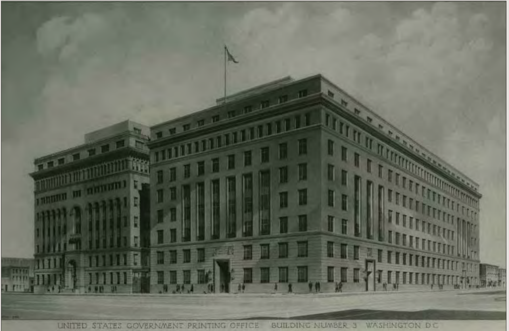
The final design removed much of the Italianate detail and, while matching the mass of Building 1, presented a more stripped down, modern appearance.
