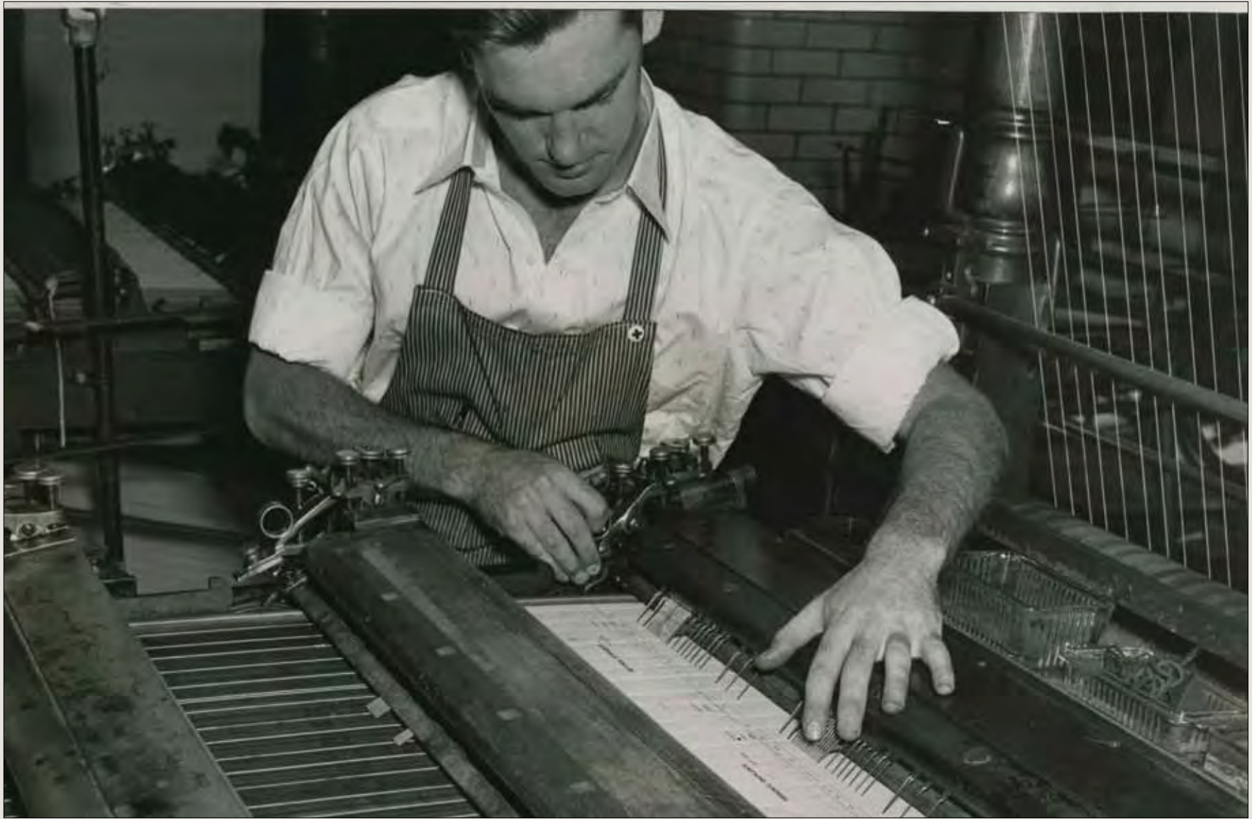
GPO produced a wide variety of lined and ruled paper and record books, as well as lined and ruled forms. Here an apprentice adjusts the pens of a ruling machine which applied the pale red and blue lines.
