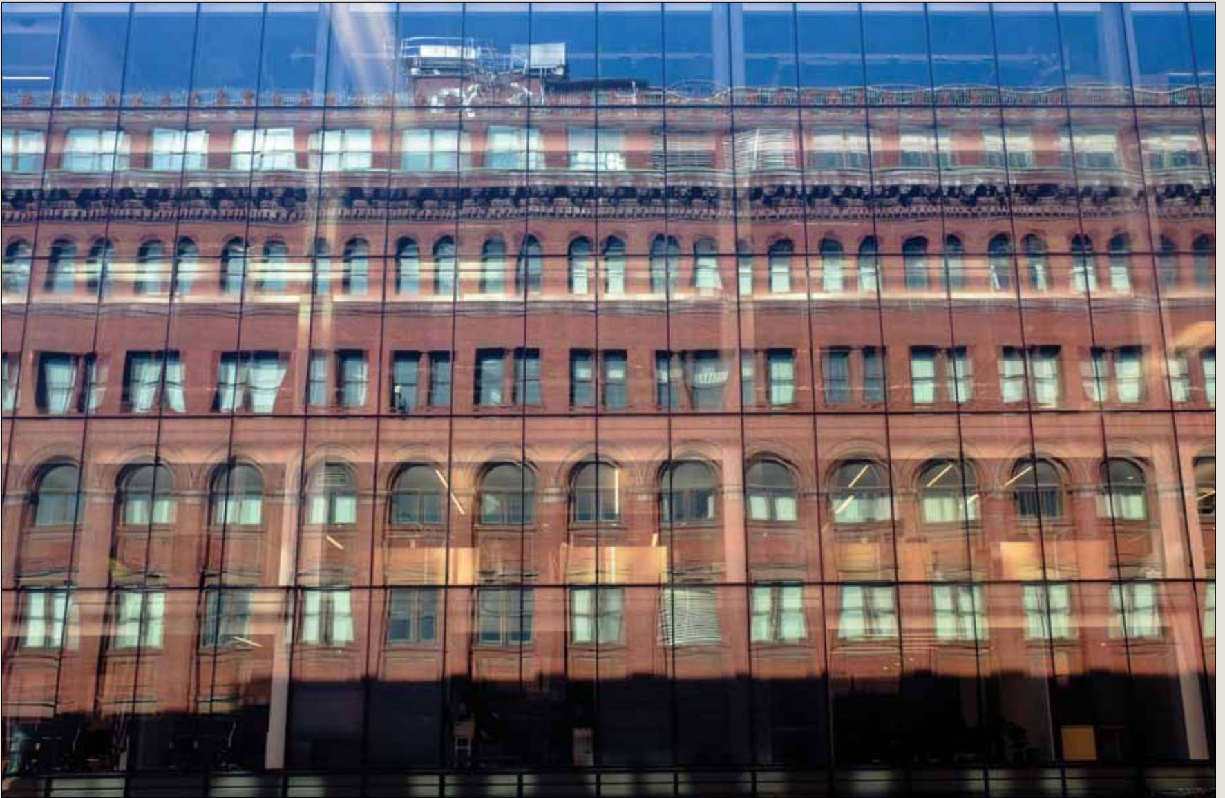
Building 1 reflected in the glass of its new neighbor across G Street NW in 2016.
