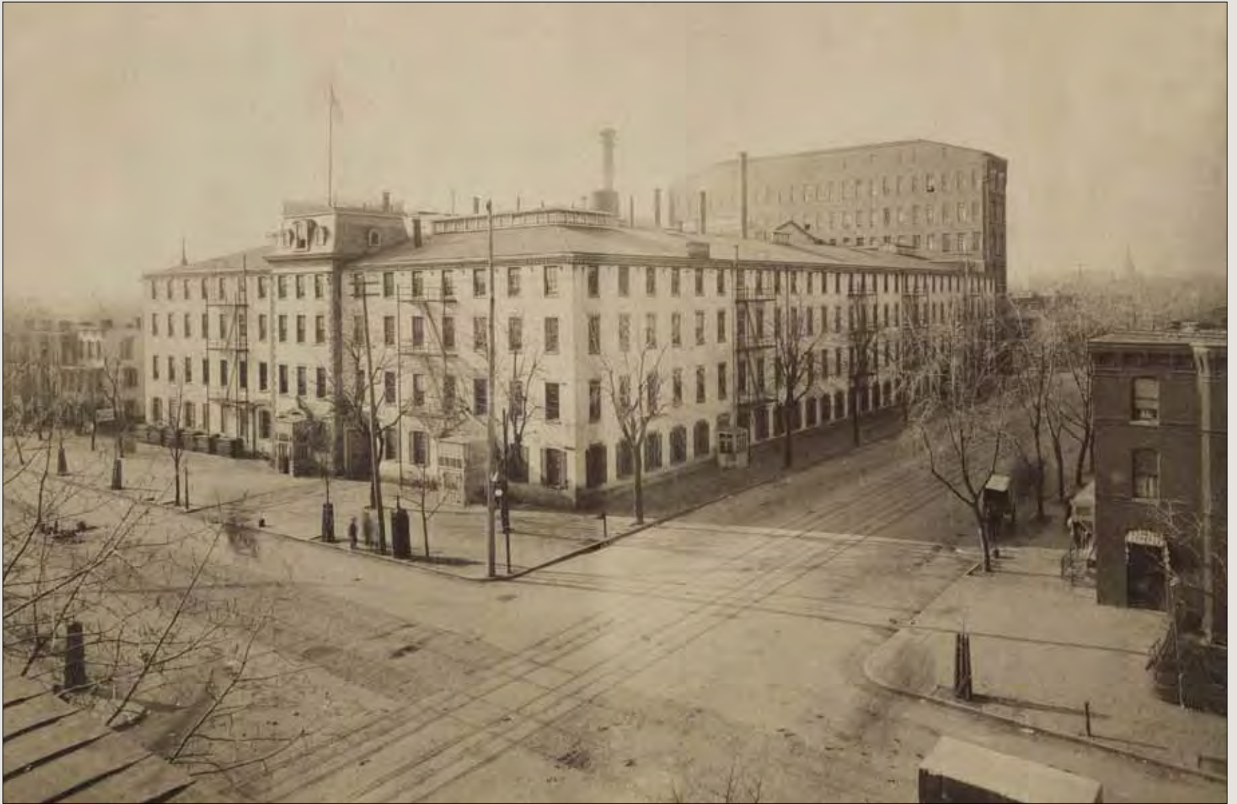
GPO continued to grow. By 1900 the inner courtyard had been built in, and in 1896 an annex had been built across the rear, eight stories tall, but very narrow. The photo shows that the neighborhood had become a residential district of modest row houses and small businesses.
