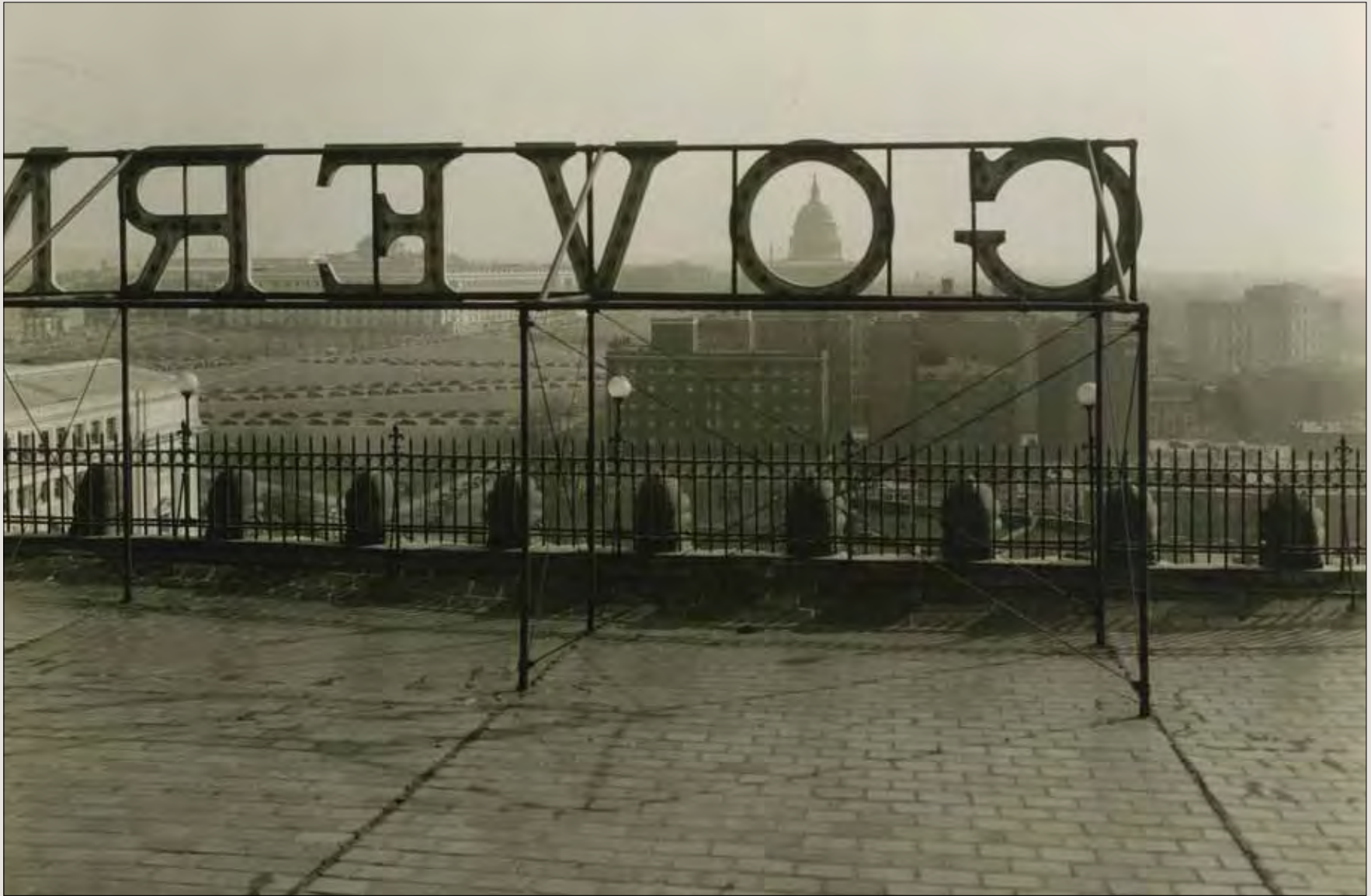
Another of the features of the 1922 renovation was a roof terrace where employees could relax or eat lunch, behind the agency's electric sign.
