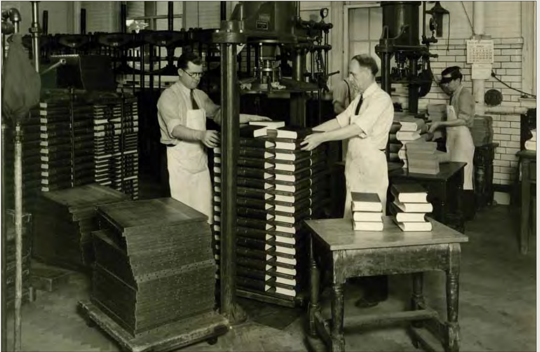
In this photo from the 1930s, newly cased-in books are packed between brass-edged boards in a hydraulic press that assures that the book will remain unwarped.
