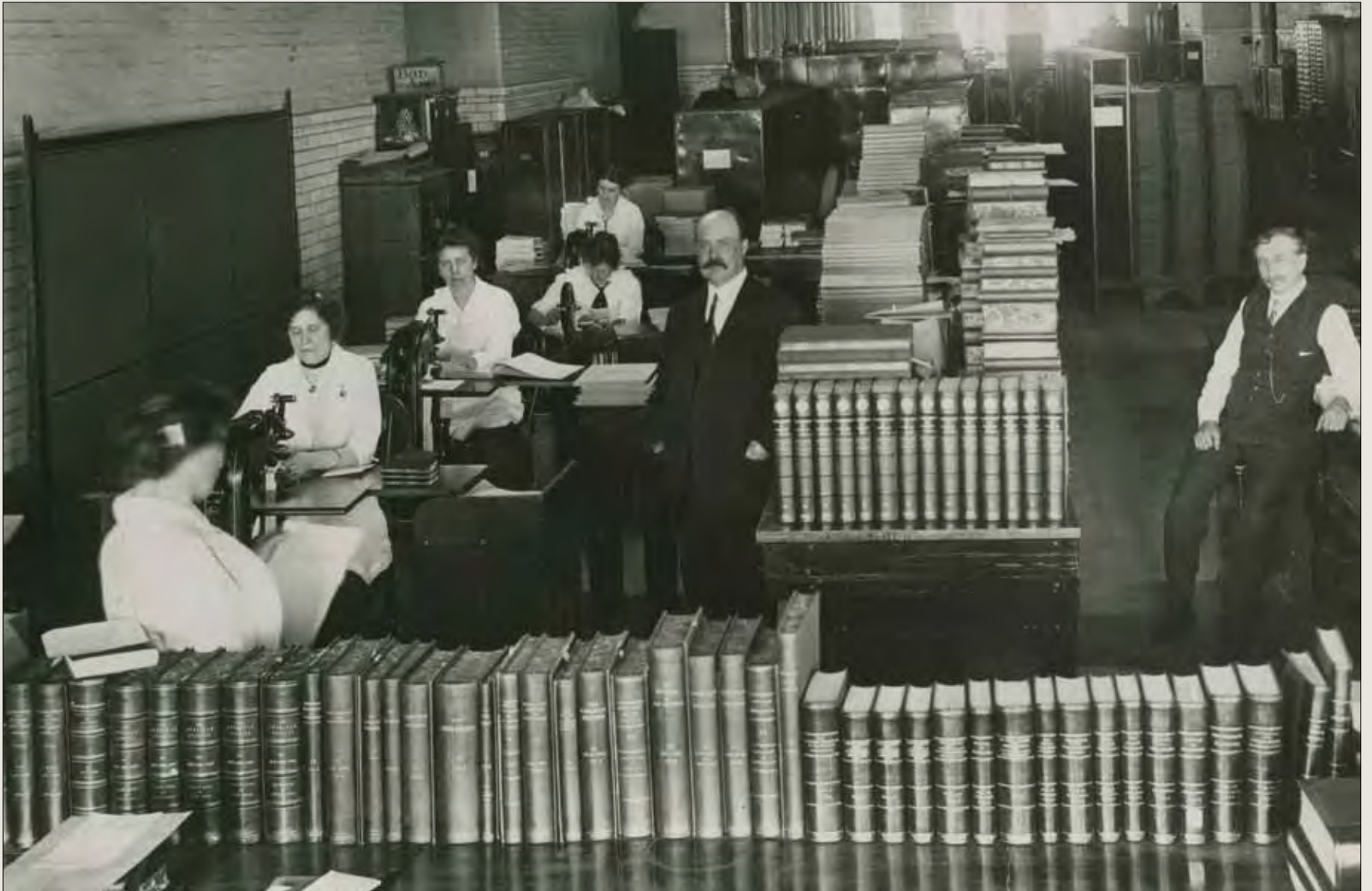
The Bindery has been home to many interesting machines. These women are “indexing” in this photo circa 1910, which in binding terms means cutting the notches known as thumb indexes into the book’s fore edge.
