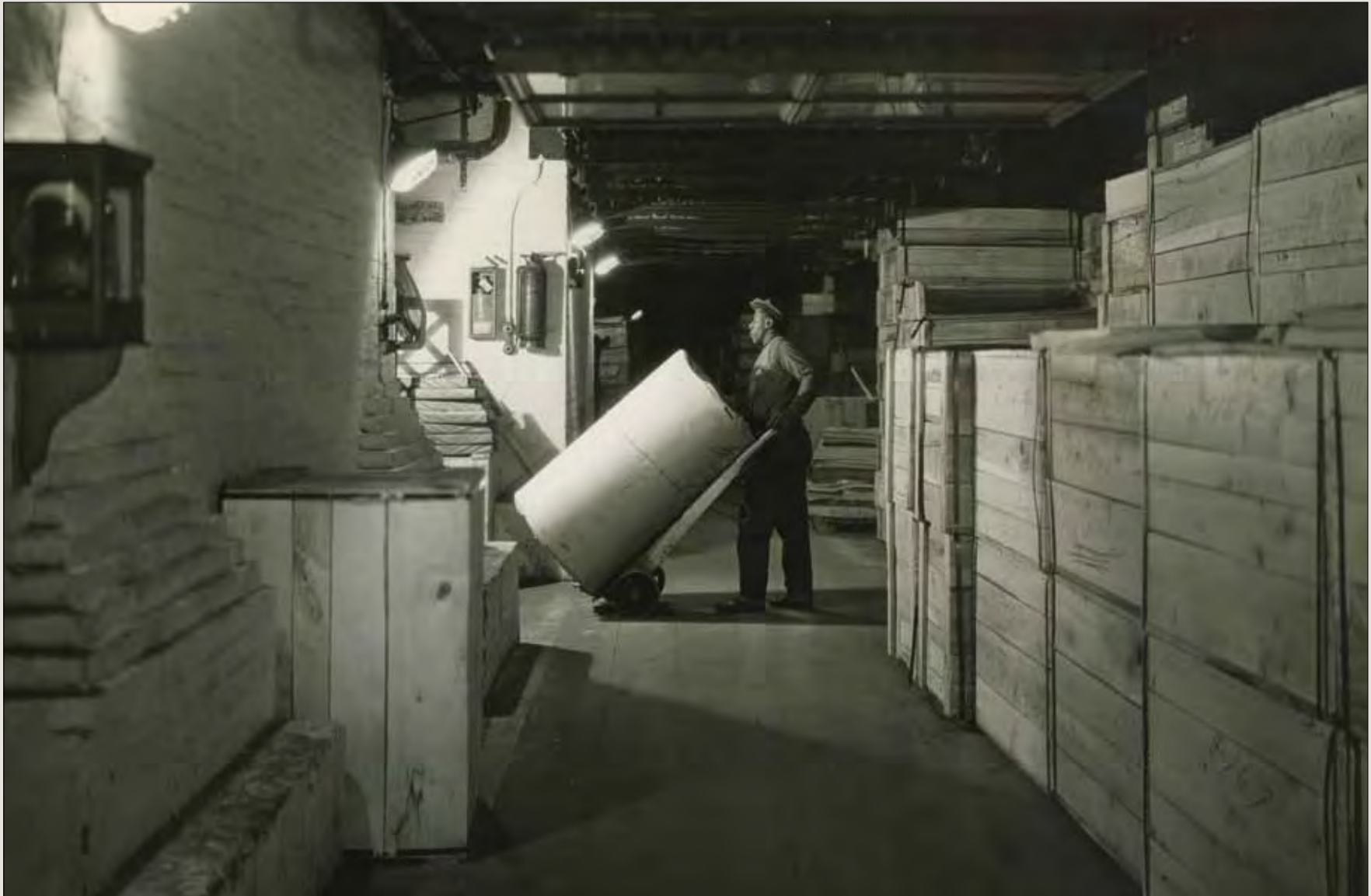
In the days of GPO's greatest output, every nook and cranny was utilized. Here paper is stored in the basement of Building 1 during the 1930s. Two of the massive pylons that support the building are visible at left.
