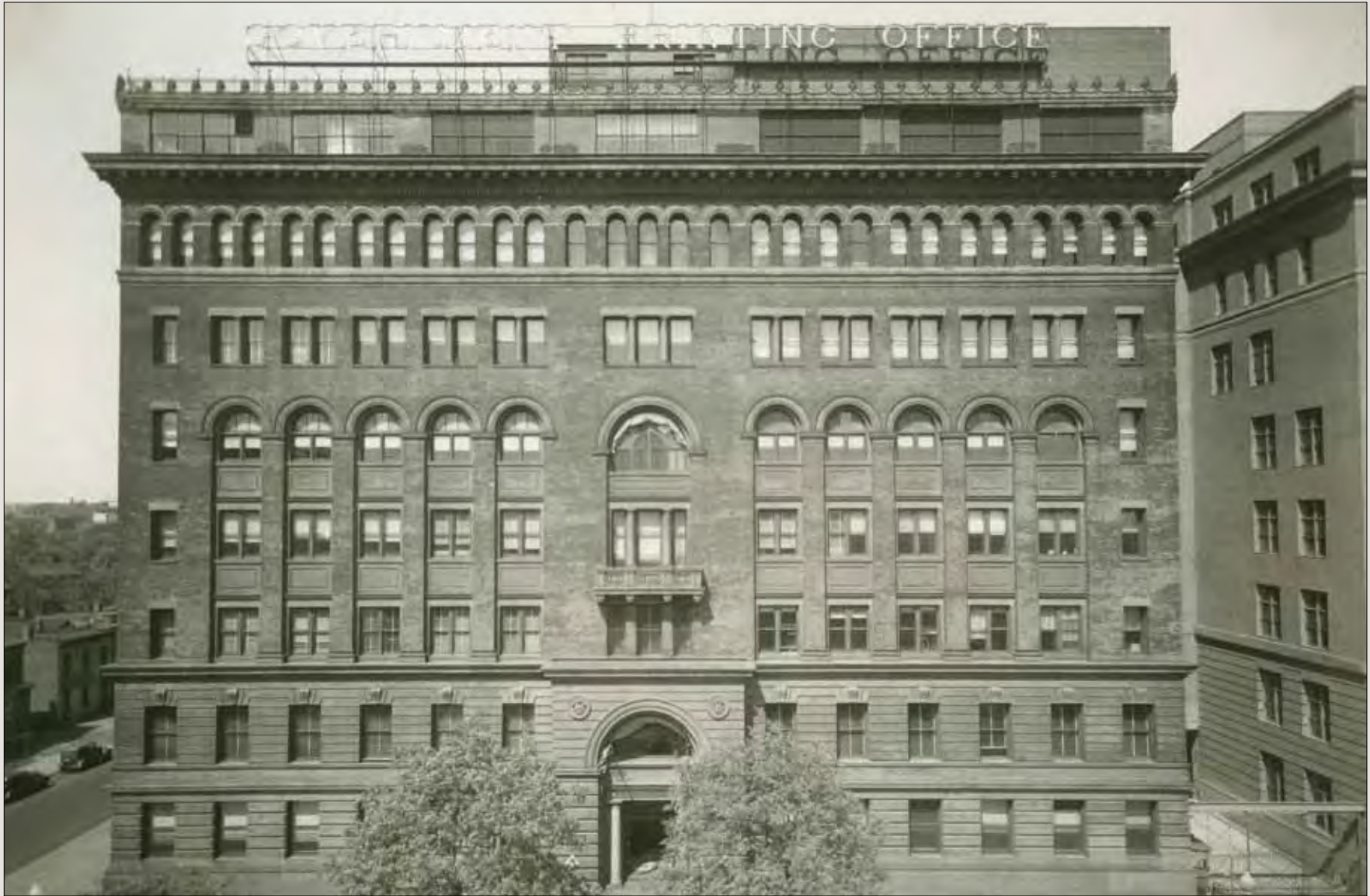
The North Capitol Street front of Building 1, with the raised roof of Harding Hall visible upper right, circa 1940. The electric sign proclaimed GPO's location from the 1920s until 1960.
