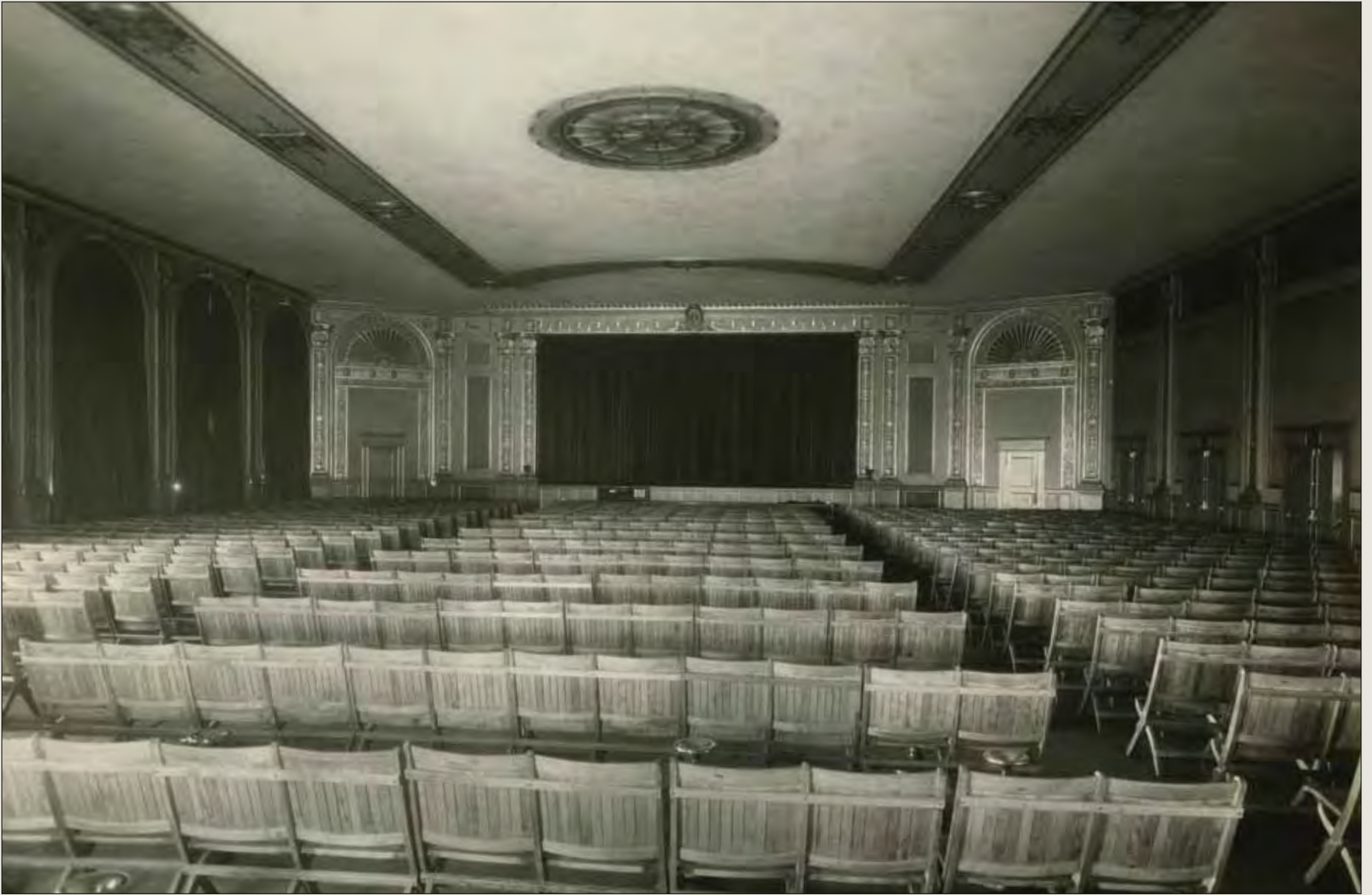
Harding Hall was renovated in 1930. The ceiling was raised again, and a fully rigged stage was added . . .
