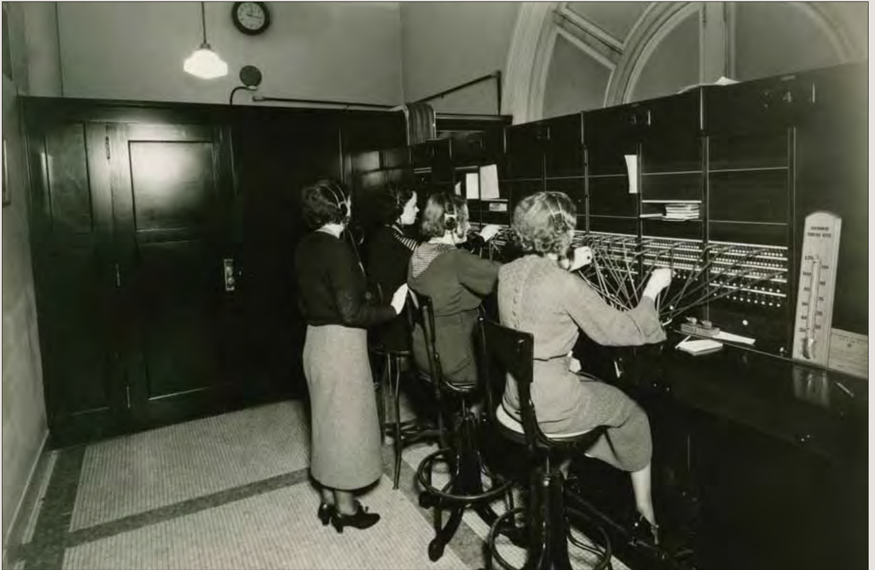
GPO installed its first telephones in the 1890s, and the first known telephone directory was a tiny folder measuring 3" x 4". Here operators run GPO's main switchboard in Building 1 during the 1930s.
