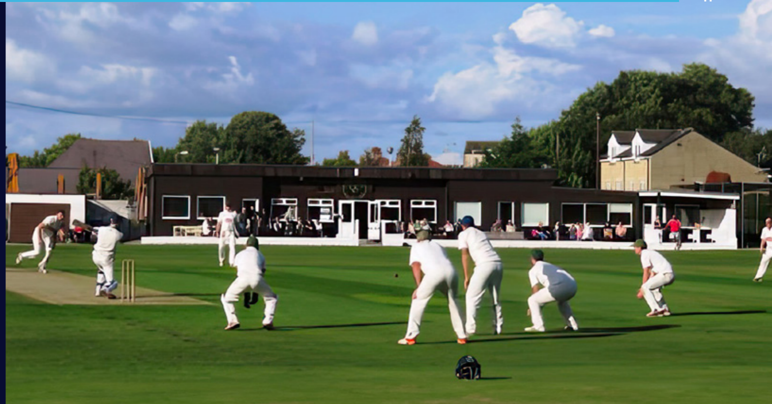
The club before external insulation was fitted. Photo credit: Carnforth CC, Lancashire.
