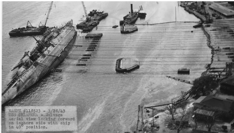
Righting the capsized Oklahoma was a major effort requiring shore winches. Source: U.S. Navy.
