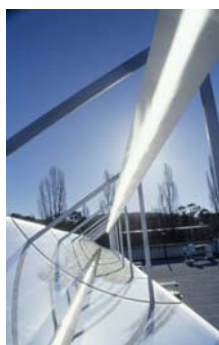
CHAPS system installed at ANU
