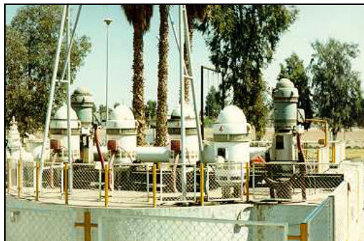
Figure 78: Pumping Plant No. 1 (Nov 1986)
