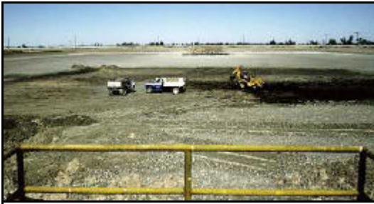
Figure 155: Cleanout of one of Mexicali's sewage treatment lagoons (Nov 1994)
