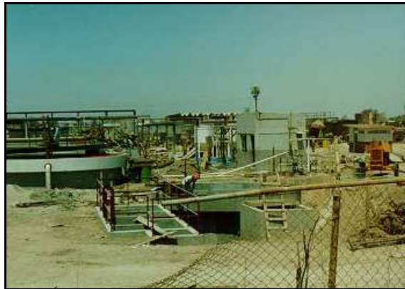
Figure 84: Construction of treatment works at Quimica Organica (Jul 1987)
