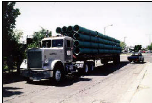
Figure 179: PVC pipe being delivered for sewer line replacement (Apr 1995)
