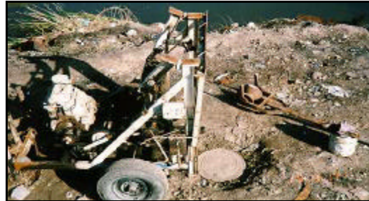
Figure 156: Sewer cleanout underway at Av. Reforma (Nov 1994)
