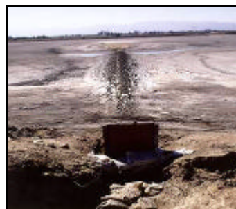
Figure 147: A primary treatment lagoon drained to repair distribution system (Aug 1994)
