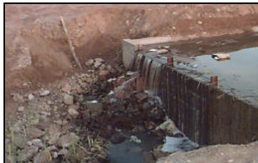
Figure 206 - Alamo River weir (Jan 1998)
