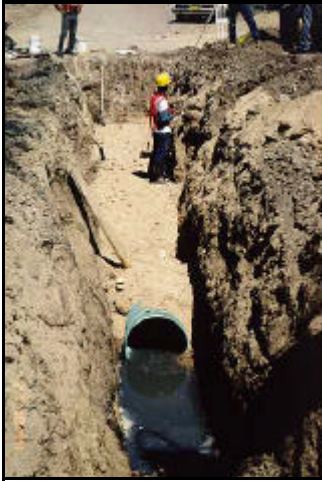
Figure 178: Replacement of concrete pipe with PVC pipe (Apr 1995)
