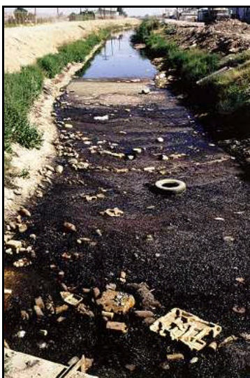
Figure 166: Mexicali Drain at Highway 2 crossing (Apr 1995)
