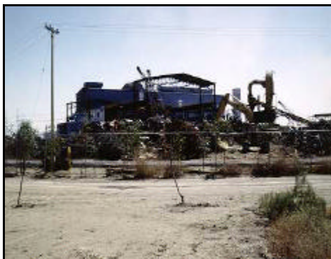
Figure 151: Siderurgica California, a steel recycling plant (Oct 1994)
