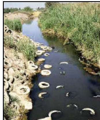
Figure 143: Bypass of raw sewage from Gonzalez-Ortega (Aug 1994)
