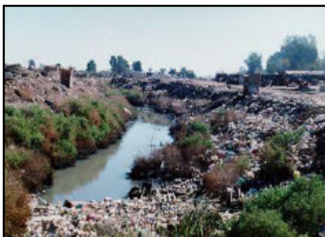
Figure 159: Mexicali Drain at San Felipe Highway crossing (Feb 1995)
