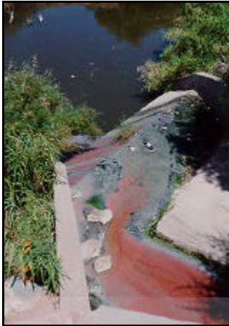
Figure 170: Raw sewage discharging to New River via storm drain (May 1995)
