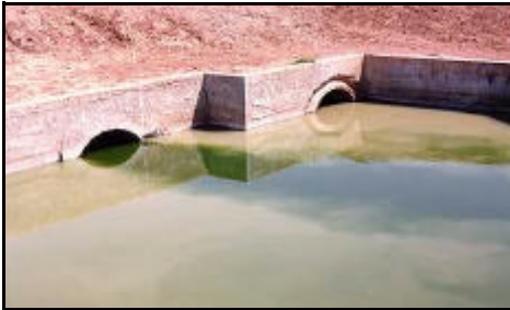
Figure 89: Color difference in effluent from Mexicali lagoons indicates disparity of treatment in lagoon cells (Apr 1988)
