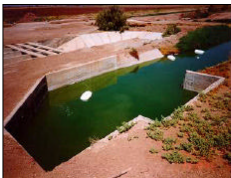
Figure 117: Effluent from treatment lagoons--treatment effectiveness is much better during warmer months (Jul 1991)
