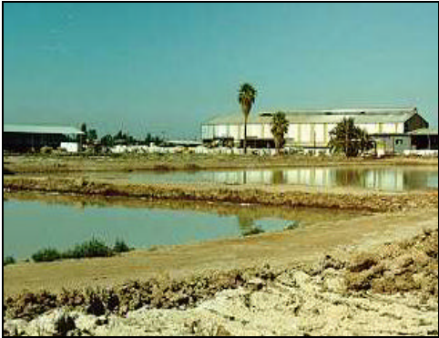
Figure 85: Wastewater basins at Fabrica de Papel S.F. (Jul 1987)
