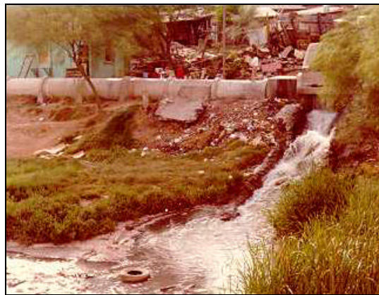
Figure 41: Raw sewage bypass from North Collector to Drain 134 (May 1978)
