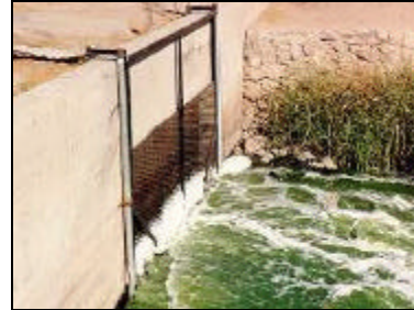
Figure 104: Screen to reduce foam at Mexicali effluent outfall to New River (Jul 1989)
