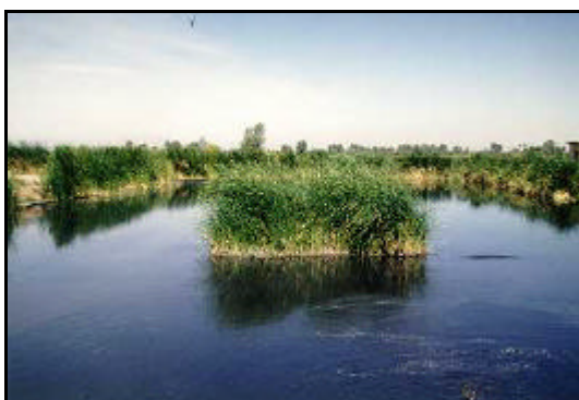
Figure 168: Gonzalez-Ortega sewage treatment lagoons (Apr 1995)
