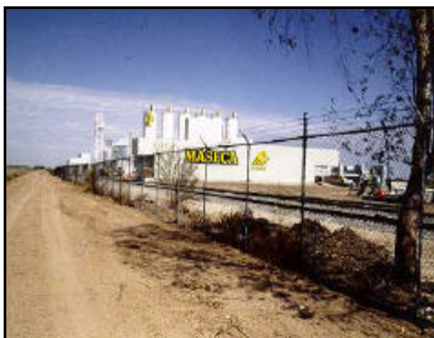
Figure 153: Maseca, a food processing plant (Oct 1994)
