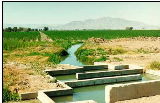
Figure 81: Distribution system for effluent irrigation from Mexicali sewage treatment lagoons (Mar 1987)
