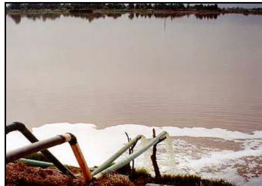
Figure 135: Mexicali sewage treatment lagoons (Apr 1994)
