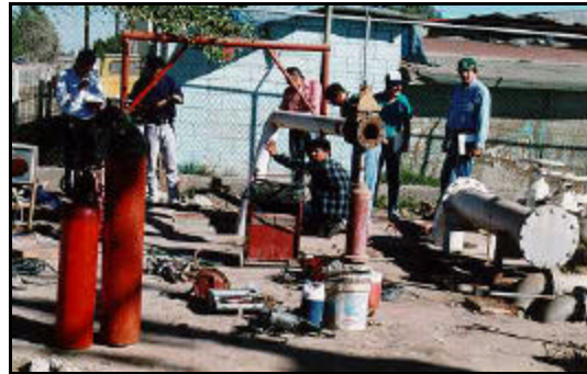
Figure 157: Repairs underway at Gonzalez-Ortega pumping station (Feb 1995)
