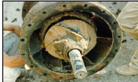
Figure 90: Replacement of worn pump at Pumping Plant No. 1 as part of joint U.S./Mexico $1.2M project (Feb 1988)
