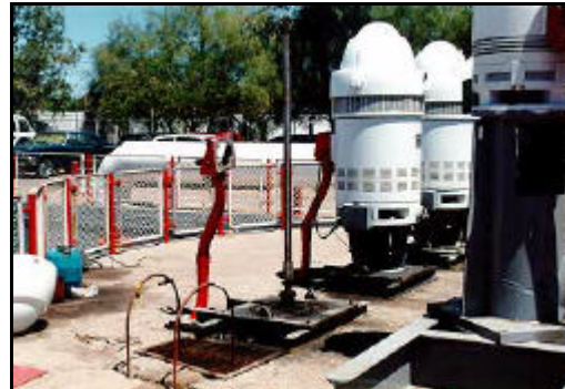
Figure 181: Repairs underway at Pumping Plant No. 1 (Apr 1995)
