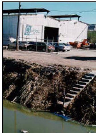
Figure 158: An opaque blue discharge from the Quipac facility (Feb 1995)
