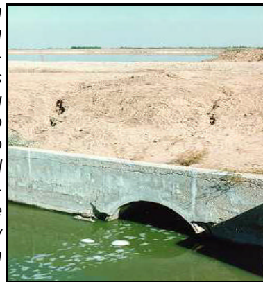
Figure 74: Effluent from Mexicali sewage treatment lagoons (Nov 1986)
