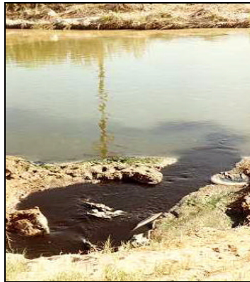
Figure 92: Raw sewage bypassing at Pumping Plant No. 2 (Oct 1988)
