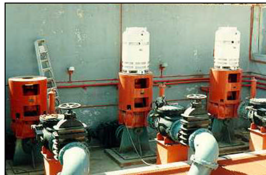
Figure 79: Pumping Plant No. 2 (Mar 1987)
