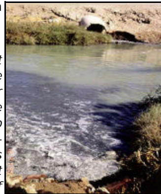
Figure 187: Bypass of raw sewage at Pumping Plant No. 2 (Oct 1996)
