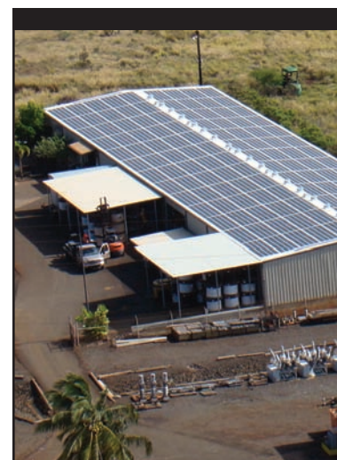
Kauai, Hawaii / Kauai Island Utility Cooperative
