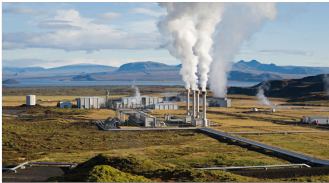
The Czech Republic's first geothermal plant, similar to Iceland's Nesjavellir plant, above, would power half the city of Liberec.
