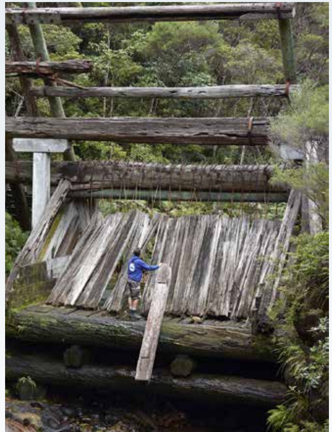
Kauri dam, built in the early 1900s to transport kauri logs from steep remote terrain to the coast.
