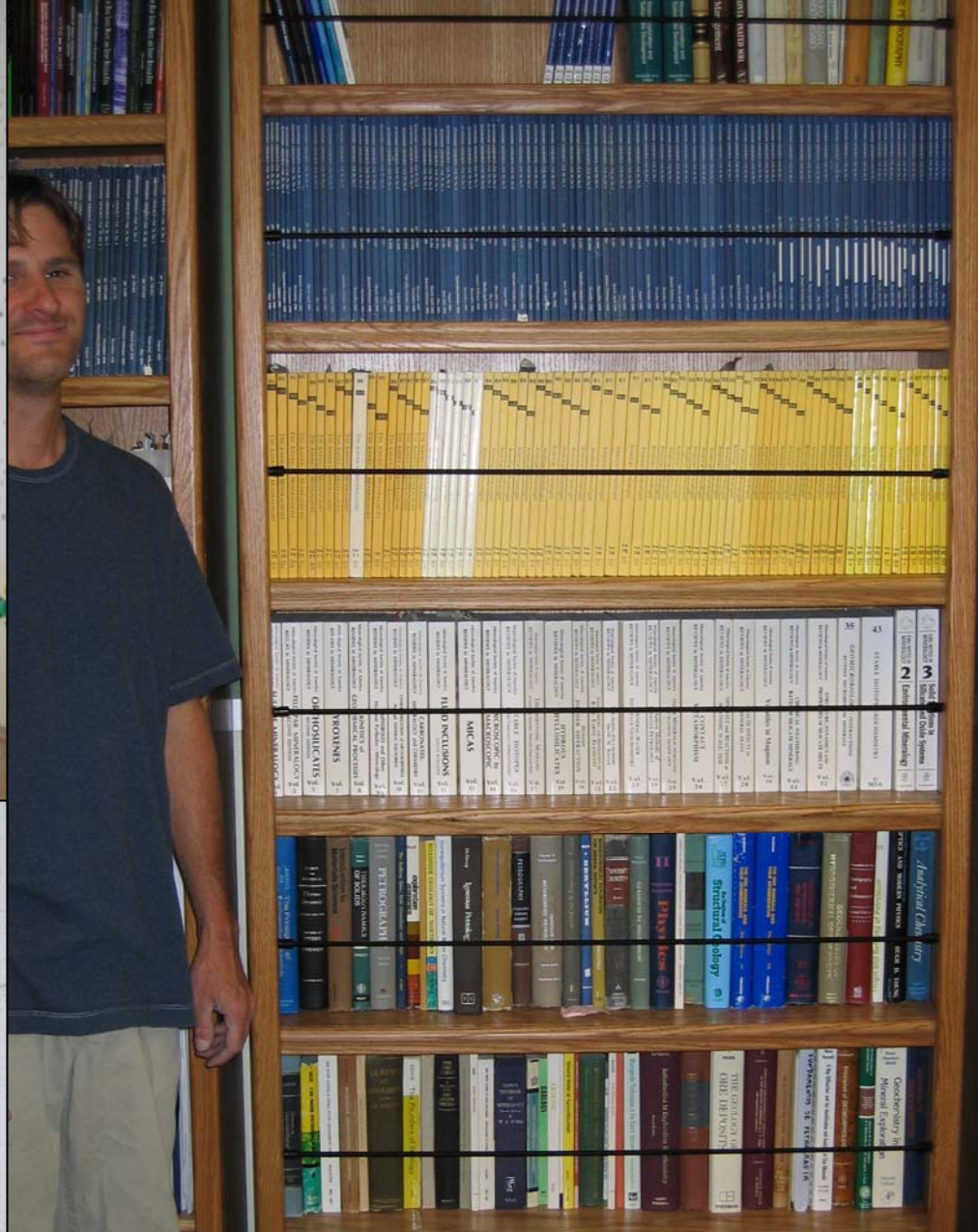
Earthquake-secure bookshelves in the office of the State Geologist
