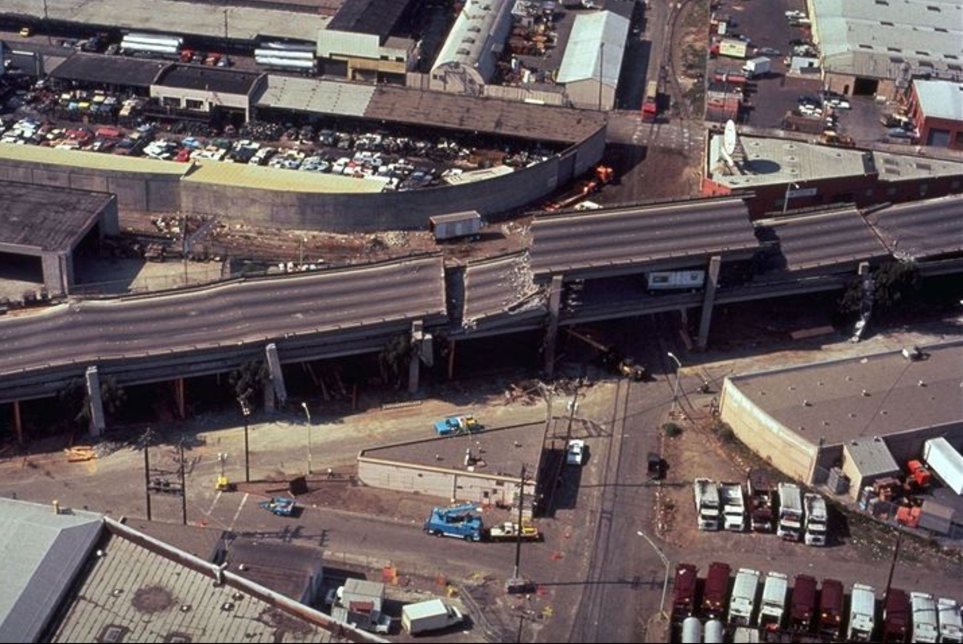
Expect damage to highways (Oakland, 1989 World Series Earthquake).
