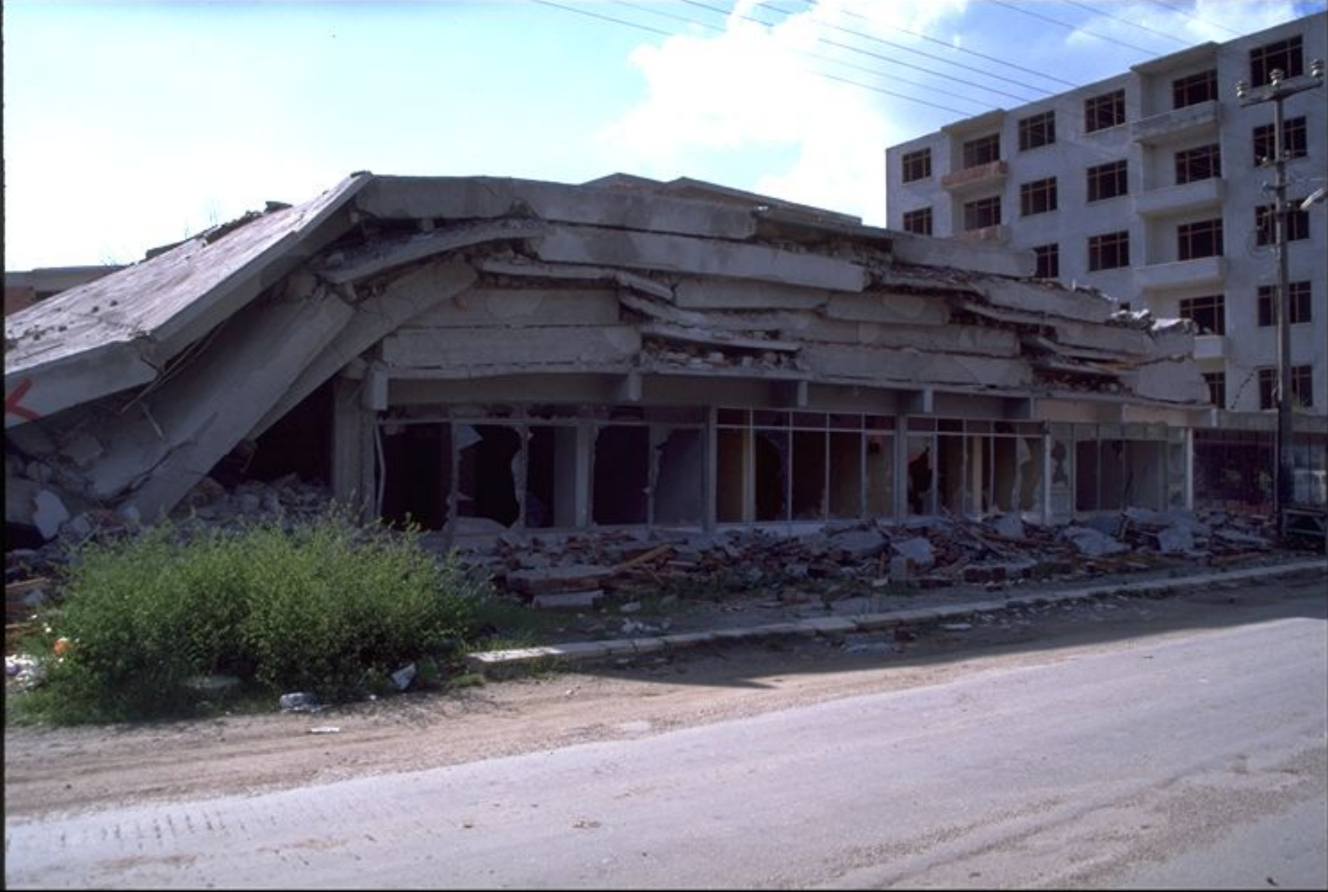
Hope that construction practices were up to code (6-story bldg, Izmit, Turkey, 1999).
