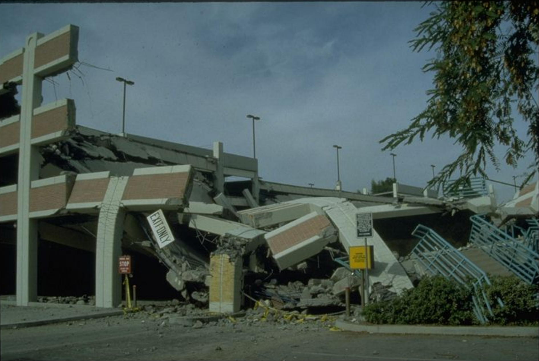
Expect problems with unusual construction (Cal State Northridge parking structure, 1994).
