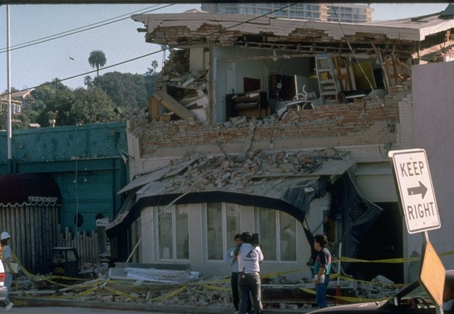
Expect damage to unreinforced masonry buildings (Northridge, 1994).
