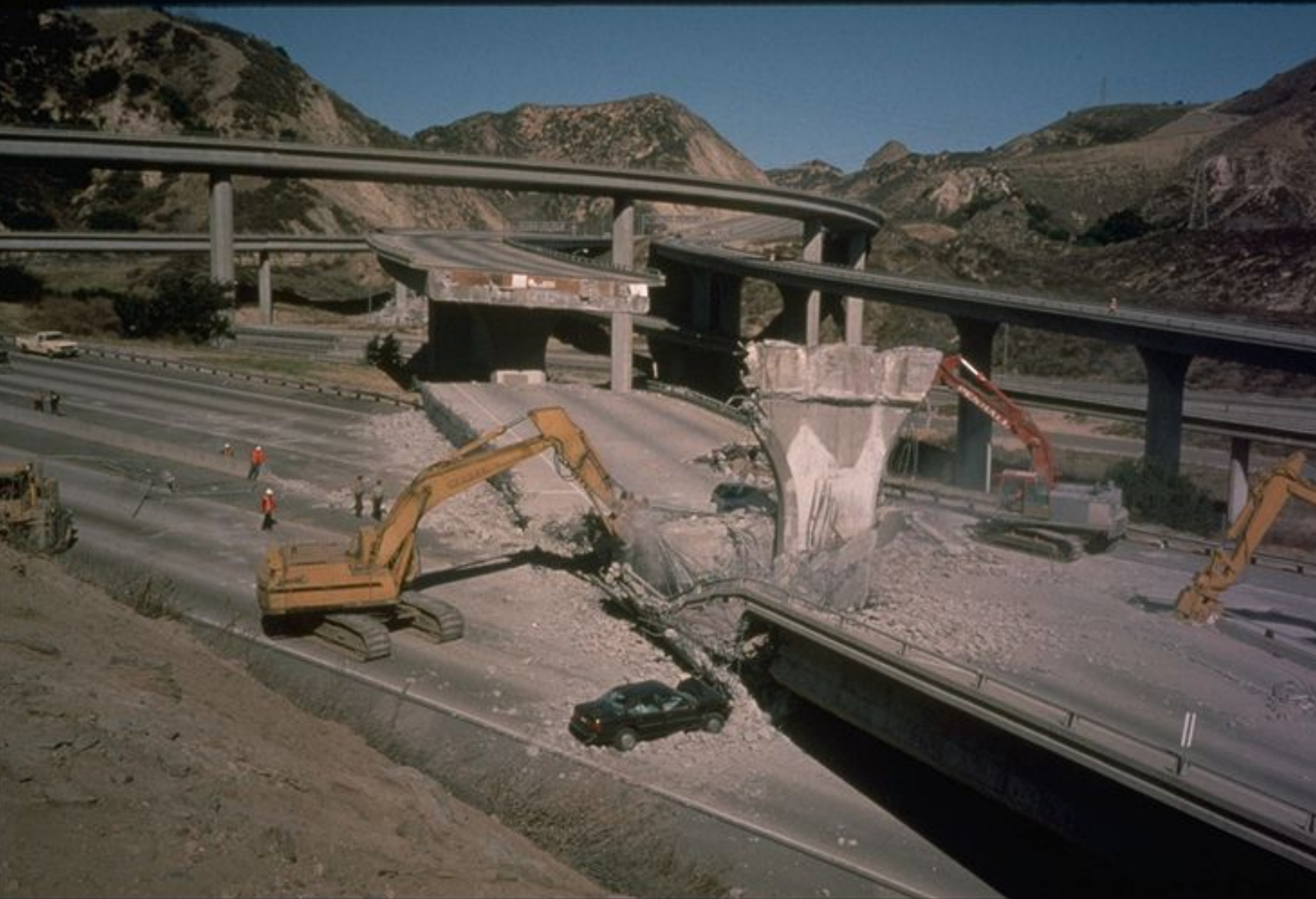
Expect damage to the infrastructure (I-5, Northridge Earthquake, 1994).
