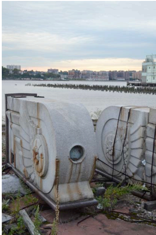
Ruins of Pier 54
