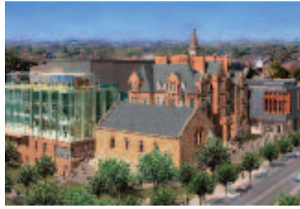
Proposed building addition under construction
