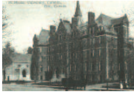
Building prior to RCM occupancy
