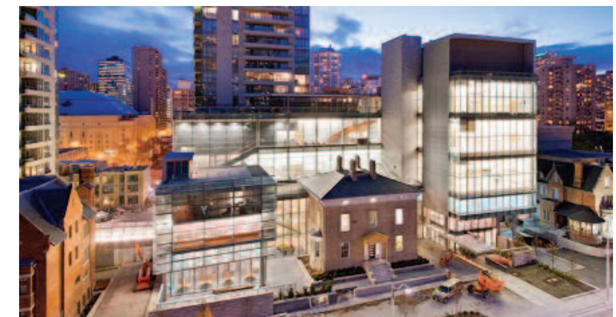
2007 View above Jarvis Street
