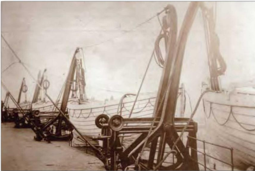
■ (Above) These deck plans show the first five watertight compartments of the Titanic that were flooded, forepeak to Boiler Room Number 6. (Below) This view of the boat deck, portside aft, shows the arrangement of Welin double-acting lifeboat davits in two sets of four. – Images courtesy of Anova Books from The Titanic Pocket Book .
