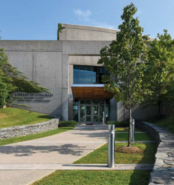
Clockwise from top: The Packard Campus for Audio-Visual Conservation; the Packard Campus data center; Laurel Howard inspects a film reel; historical film reels preserved at the Library. Shawn Miller
