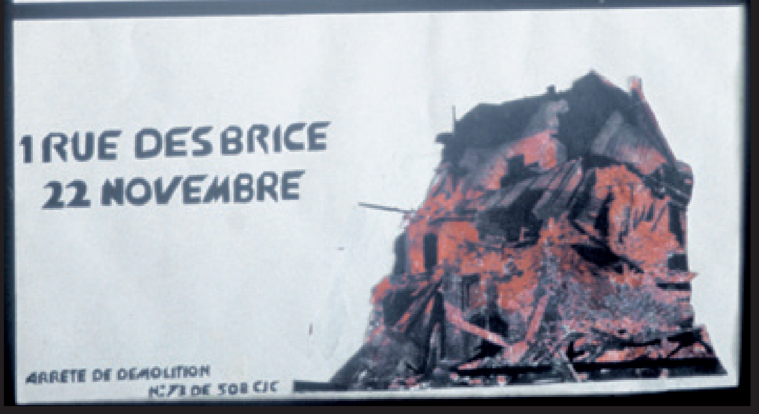
Here and on the opposite page, bottom: the students of the École des beaux-arts de Nancy developed an energetic campaign creating posters against the demolition of the Villa Fournier-Defaut throughout 1974. The campaign failed to achieve its objective, but it proved a powerful contribution to raising awareness of the value of Art Nouveau heritage among both the people and authorities of Nancy
