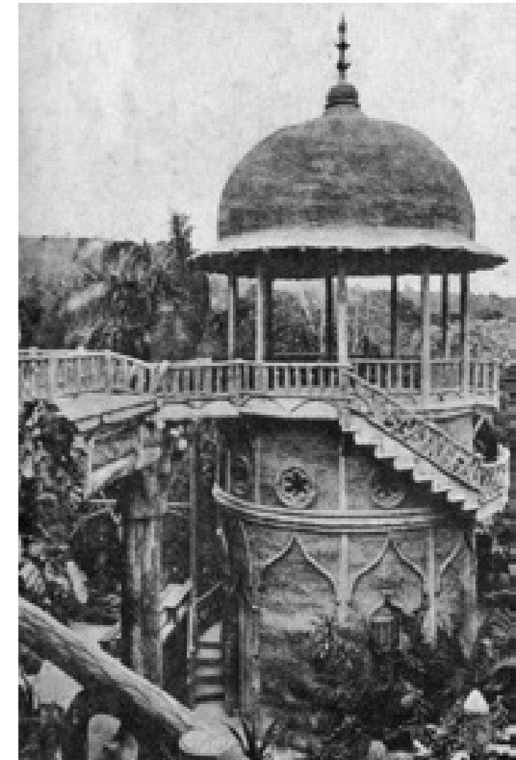
One of the towers of the Ensueño hall: All four towers were identical, each with a rather handsome reinforced concrete cupola
