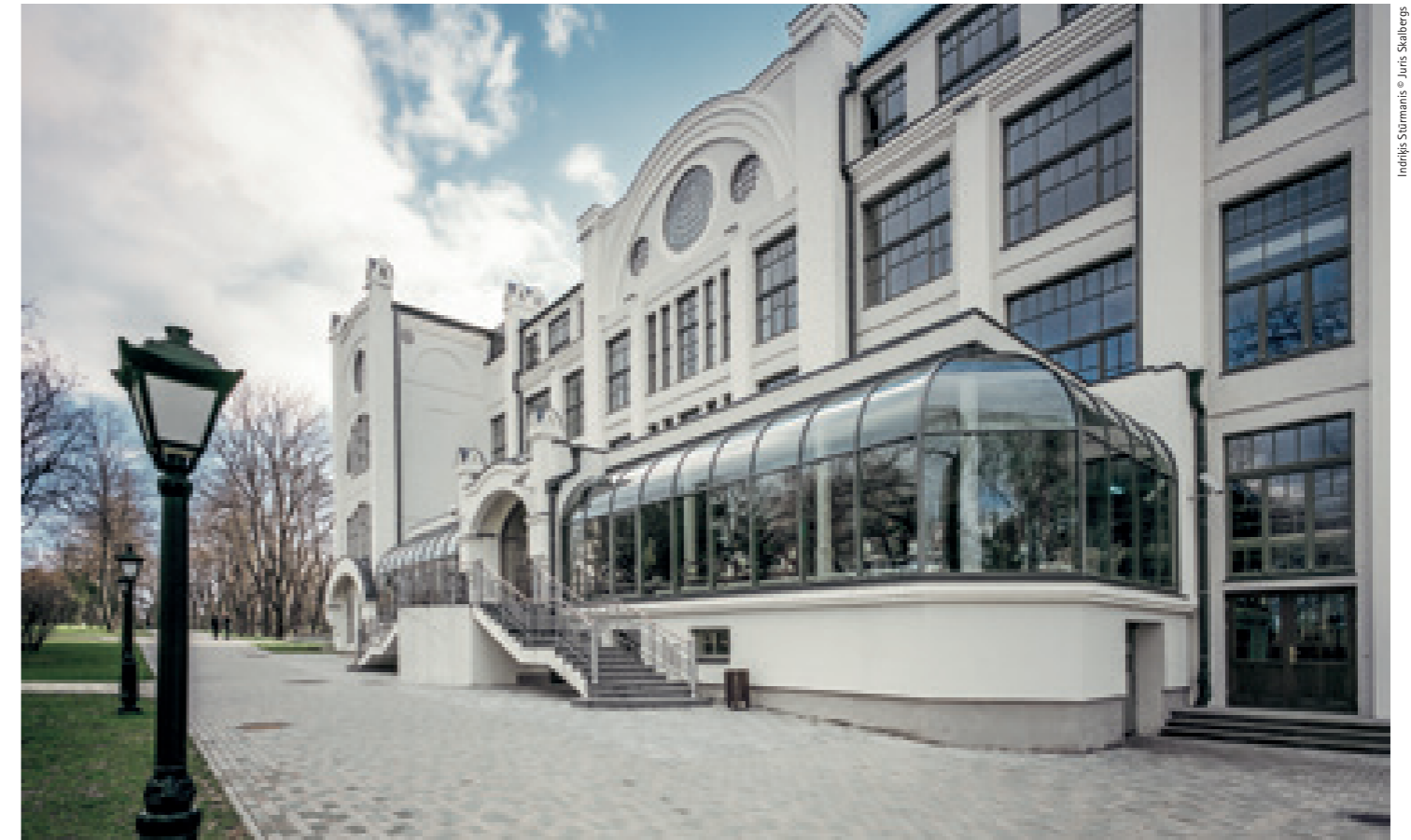
On the garden façade, the architects of the rehabilitation added a glass-canopied restaurant hall that projects the interior of the building into the park
