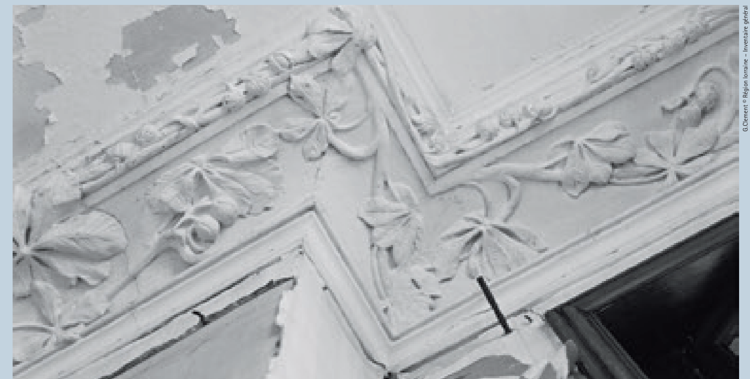
Detail of plaster ceiling mouldings, shortly before demolition in 1974 / Detall de motlures de guix del sostre, poc abans de l'enderroc el 1974
