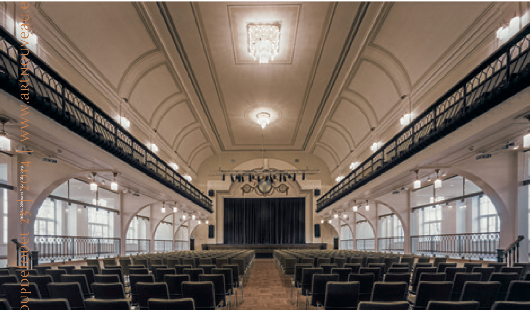
Main hall after restoration, with naturally lit side galleries and widened stage; the medallions painted over the stage were reconstructed from period photographs, like the 1939 image below
