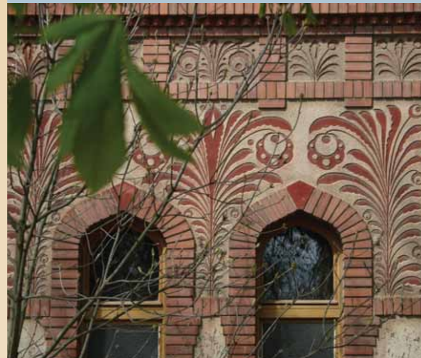
Ferenc Pfaff, 1910. Gyula, elementary school. Façade with brick stripes and sgraffito Hungarian flower motifs
