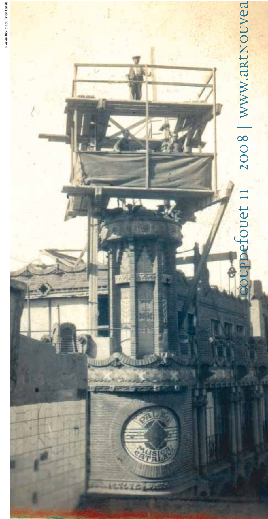
Final phase of the Palau's construction, c.1908
