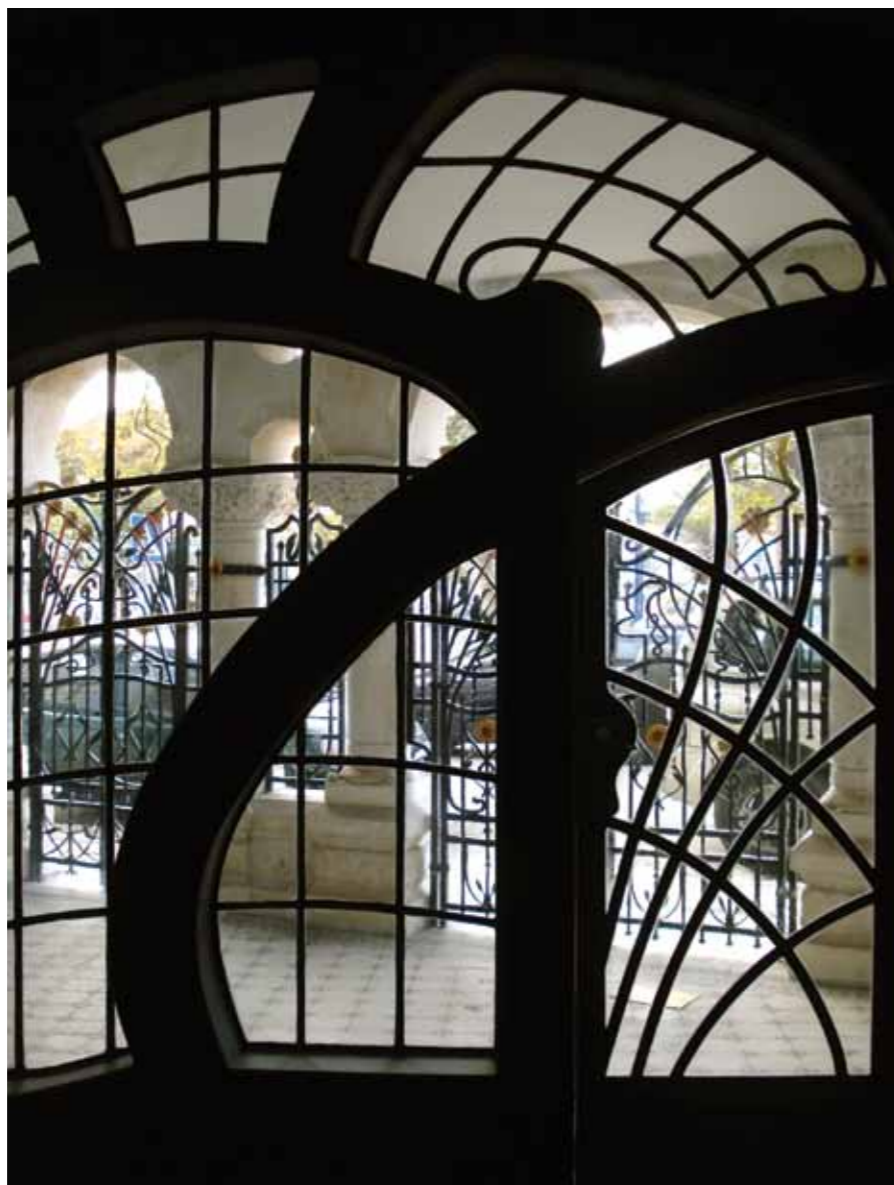
Francisco Augusto da Silva Rocha, c1907-09. Main entrance of the Casa Major Pessoa, the future Arte Nova Museum
