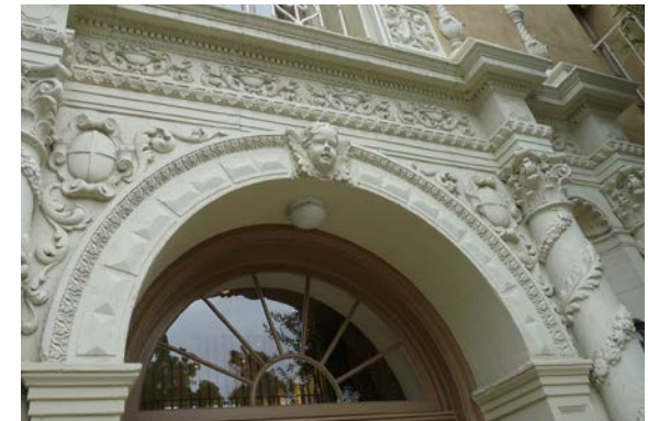
CAST CONCRETE ENTRANCE DETAIL
