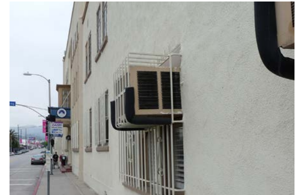
CURRENT SIDEWALK ELEVATION WINDOW AC &amp; GRILLES
