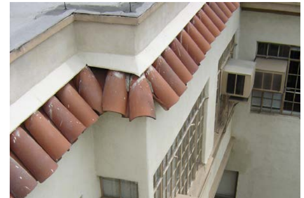
CLAY TILE ACCENT ROOFS AT THE CHEVALIER BUILDING
