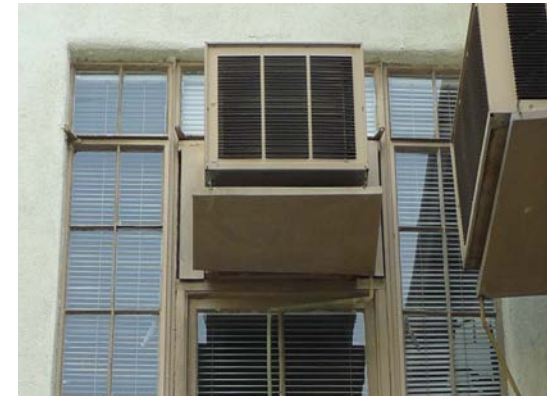
STEEL CASEMENT WINDOW WITH AIR CONDITIONERS
