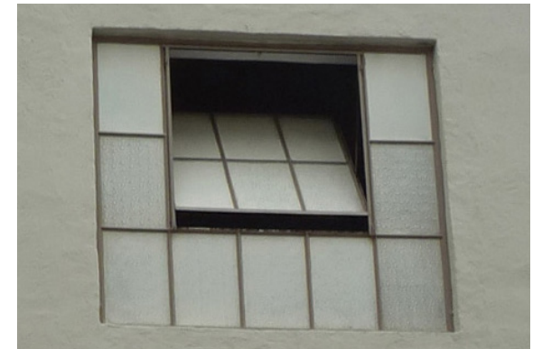
STEEL PIVOT WINDOW WITH BACK PAINTED GLASS
