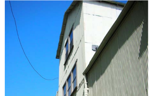
METAL ROOFING ON PRE-PRODUCTION BUILDING
