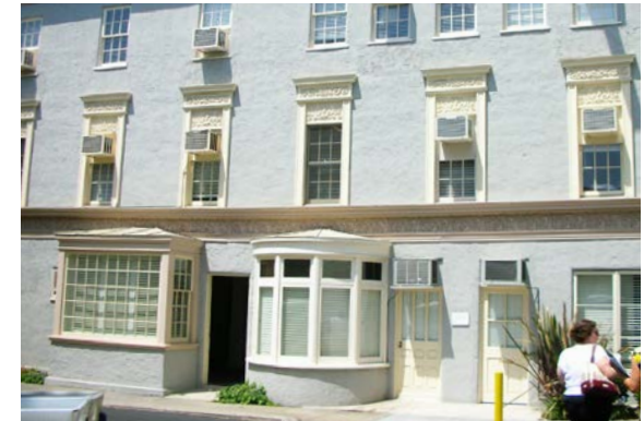
WOOD BAY AND DOUBLE-HUNG WINDOWS AT DRESSING ROOM
