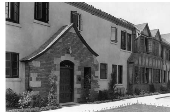
ORIGINAL WOOD SHINGLES AT ADMINISTRATION, KNOWN AS THE REDSTONE BUILDING
