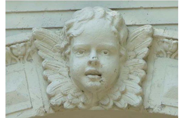
CAST CONCRETE ADMINISTRATION BUILDING DETAIL
