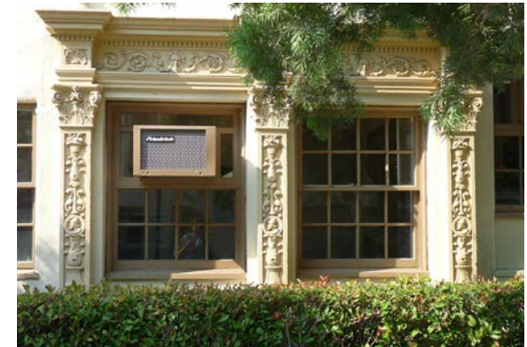
WOOD DOUBLE HUNG WINDOW IN CAST SURROUND
