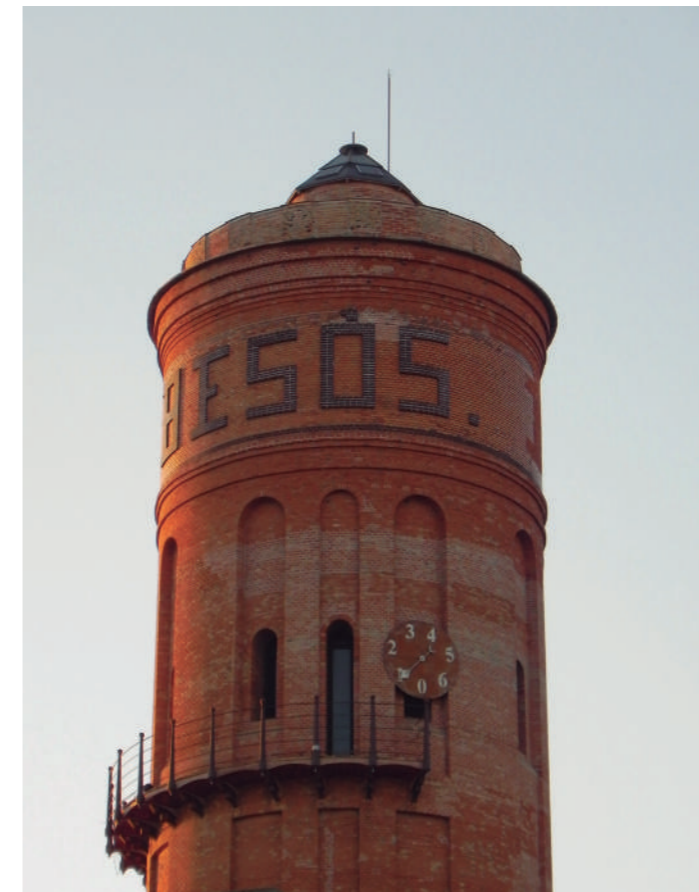
The top of the tower still preserves the original company's name and the water level measuring gauge
