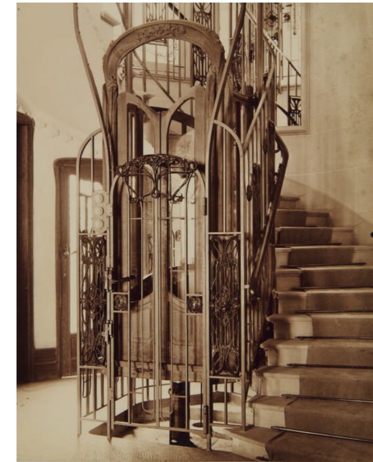
Original lift, no longer extant, in Hôtel Trémois (1909–1910) Ascensor original, avui desaparegut, de la Casa Trémois (1909–1910)
