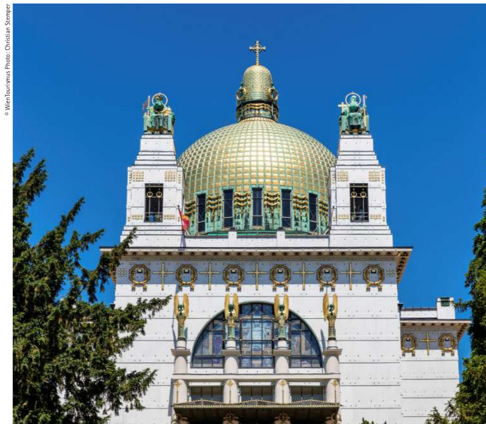
Facade of the Church of St. Leopold (1904-1907), designed by Otto Wagner Façana de l'Església St. Leopold (1904-1907), dissenyada per Otto Wagner
