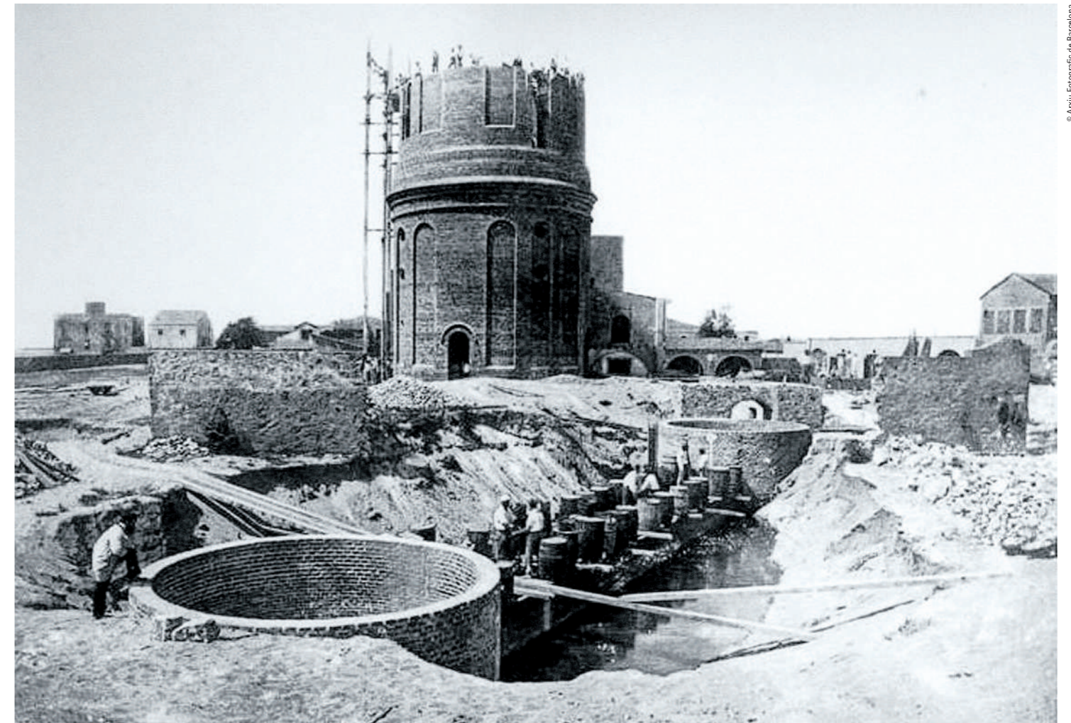
Image of the water tower's construction process in September 1880, with the collection wells in the foreground
