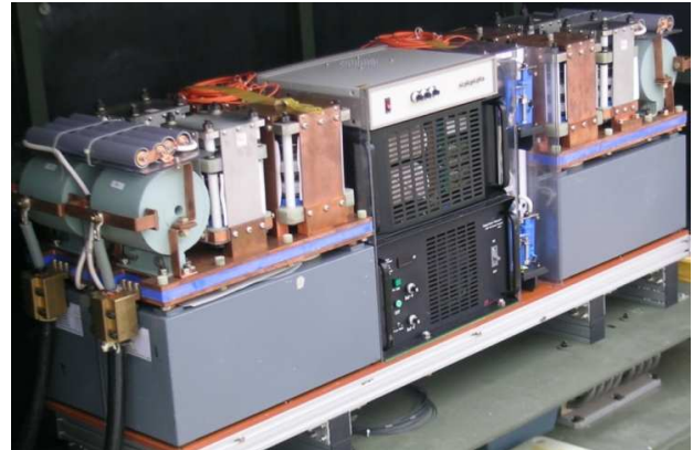
Fig. 9. Overall system of the 150 kJ CCPPS
