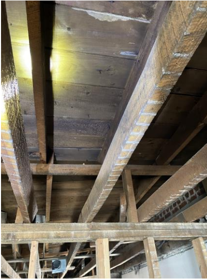
Image 10 – Existing Roof/Ceiling Framing Bearing on Interior Wall
