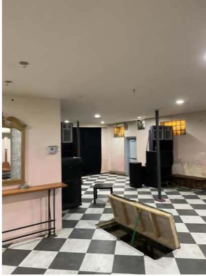
Image 21 – Main Level – Temporary Columns (Looking Southwest)
