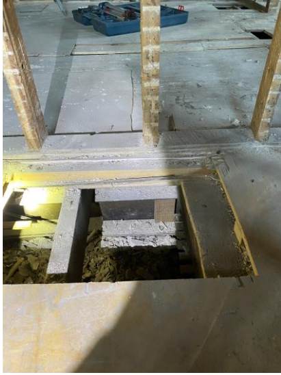
Image 18 – Second Floor – Original Steel Beam Support
