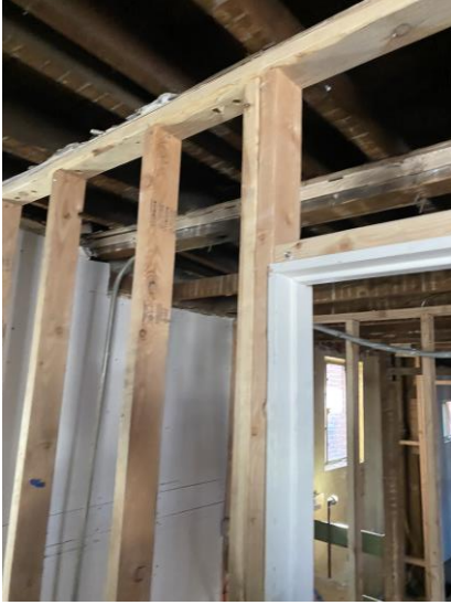
Image 12 – Altered Bearing Wall Location – Northeast Section
