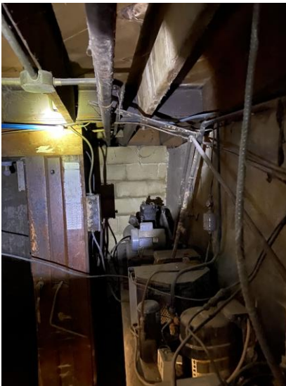
Image 23 – Main Level Framing – Modified Crawl Space/Framing
