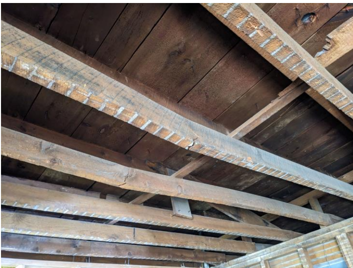
Image 14 – Overloaded Framing
