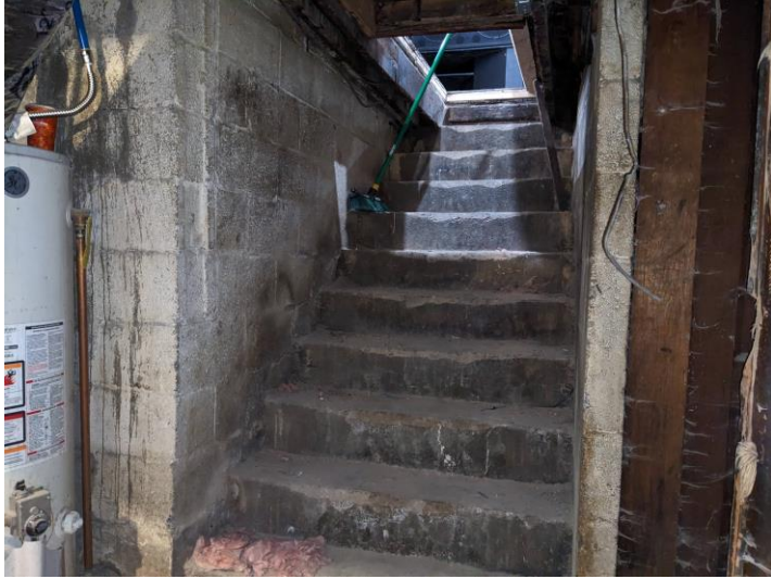
Image 28 – Crawl Space Stairs – Not Original
