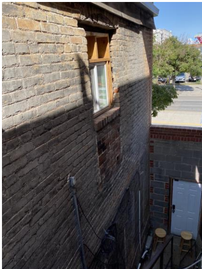
Image 5 – East Elevation (Looking North)
