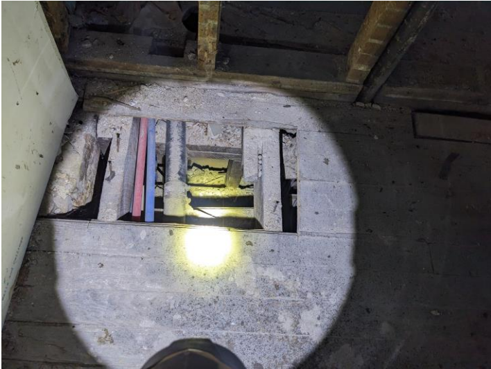
Image 17 – Second Floor – Joists Bearing on Original Wood Bearing Wall – Southeast Area
