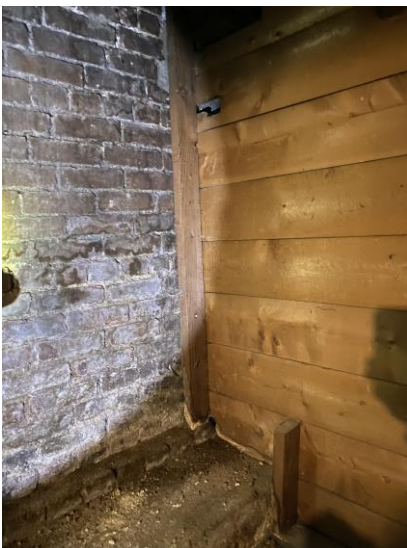
Image 24 – Crawl Space – Original Brick Foundation/Footing
