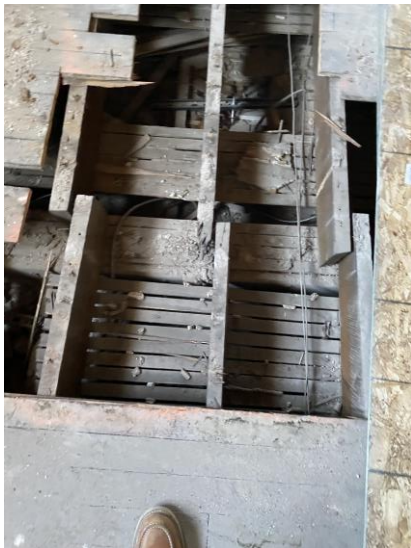
Image 19 – Second Floor – Bearing Wall Below Replaced by Beam
