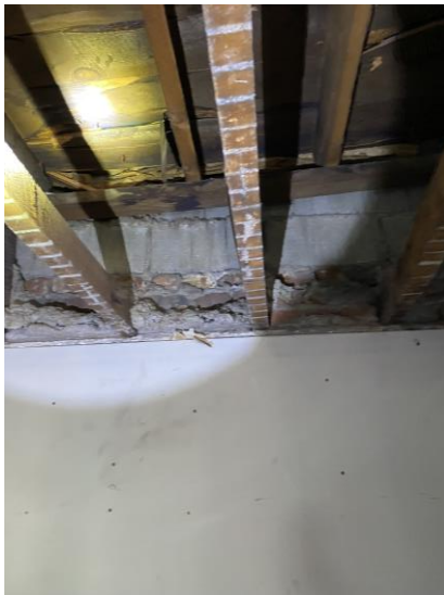
Image 9 – South Elevation – Top of Wall Past Rehabilitation
