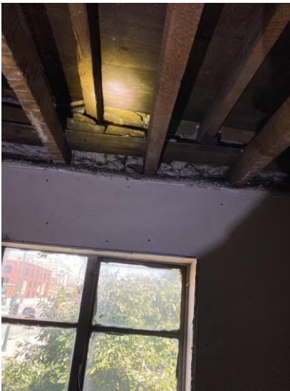
Image 11 – Existing Roof/Ceiling Framing Bearing in Brick Pockets
