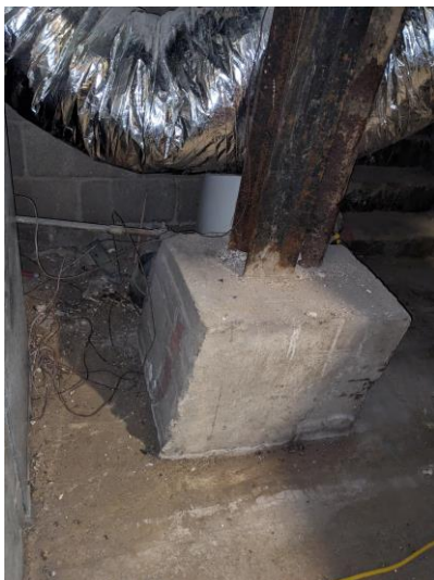
Image 27 – Crawl Space – Existing Column Support
