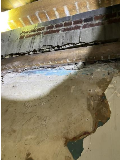
Image 8 – West Elevation – Top of Wall Past Rehabilitation
