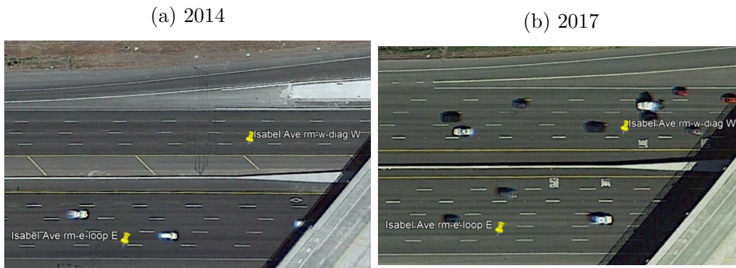
Figure 5: Lane Expansion at I-580 Express Lanes Project
