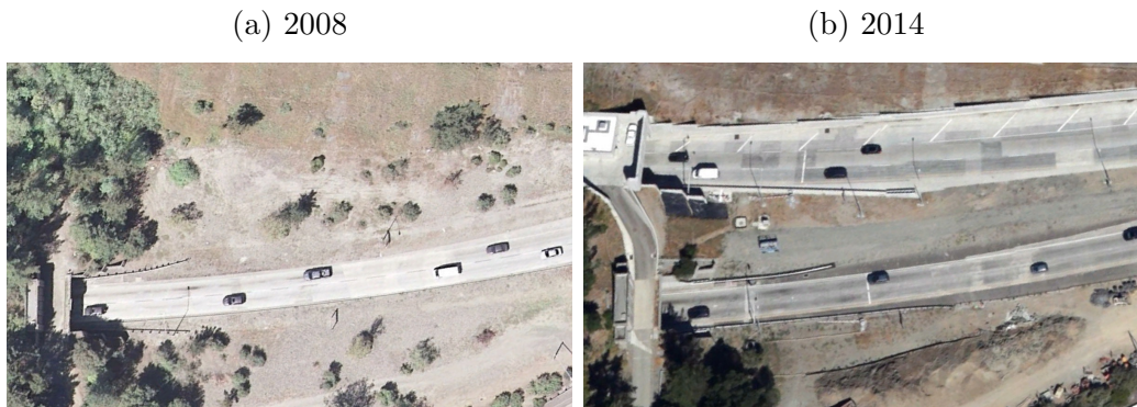
Figure 3: Fourth Bore Project at SR-24 Caldecott Tunnel
