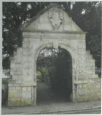
Stone arch on Station Rd
