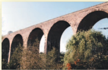
Railway Viaduct at Pensford
