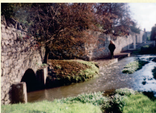
Bridge over river at Stockwood Vale
