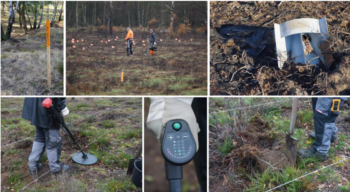
Figure 15: Clearance works. Upper row (left to right): marking of parcels, anomalies marked for excavation, find at the surface. Lower row: Detection with the “Minelab F-3 UXO”, recovery of anomalies.
