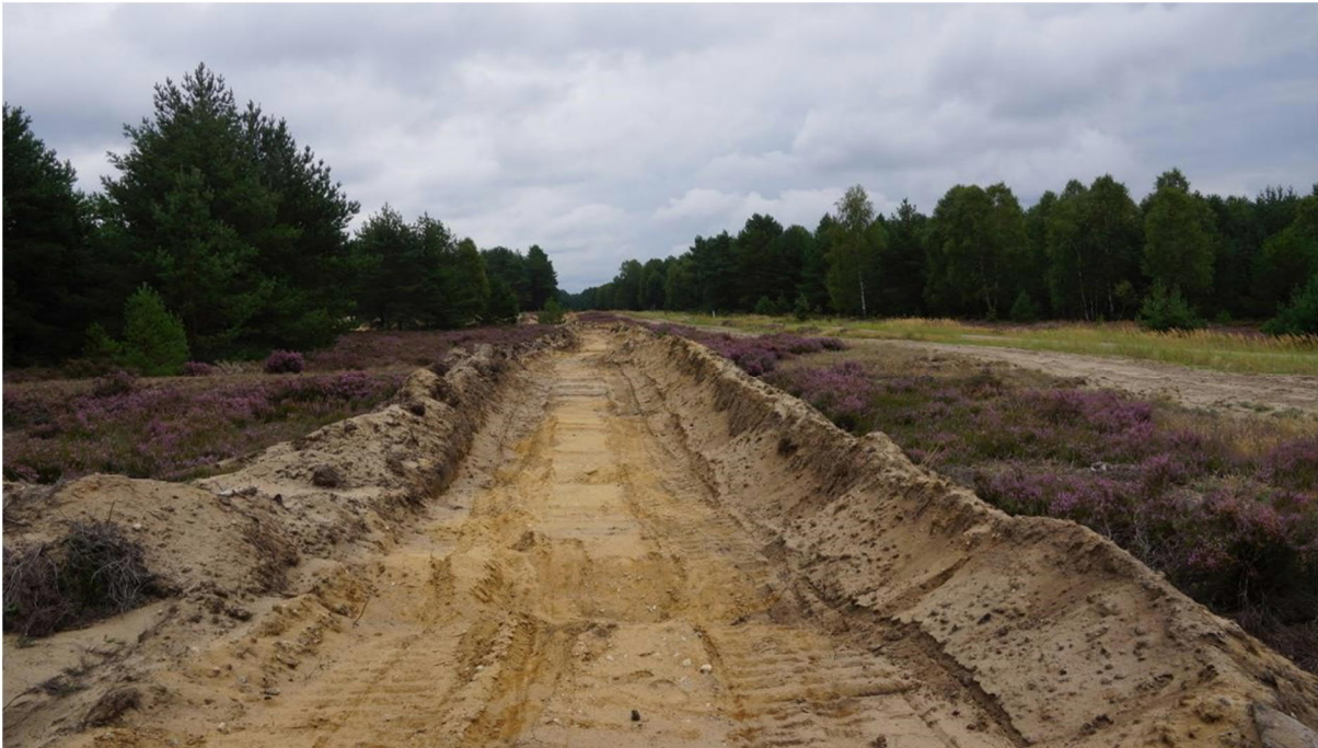
Figure 11: Fire-break as created by the remote-controlled caterpillar. For further explanations, see text.
