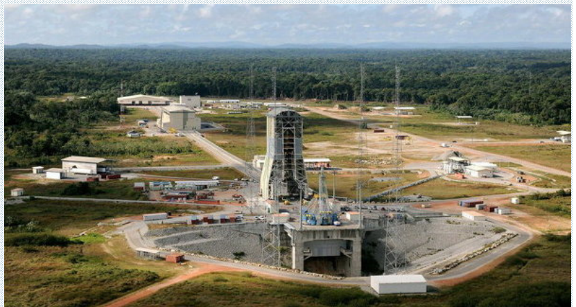
Soyuz launchpad in construction in early 2010. (credit ESA/CNES)
