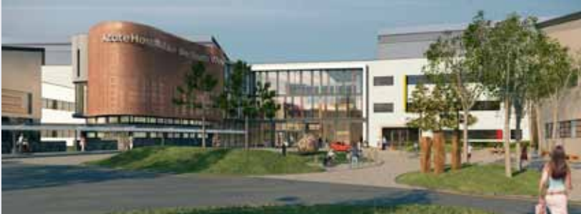
The new acute hospital for the south-west of Northern Ireland, outside Enniskillen, due to open in June 2012.
