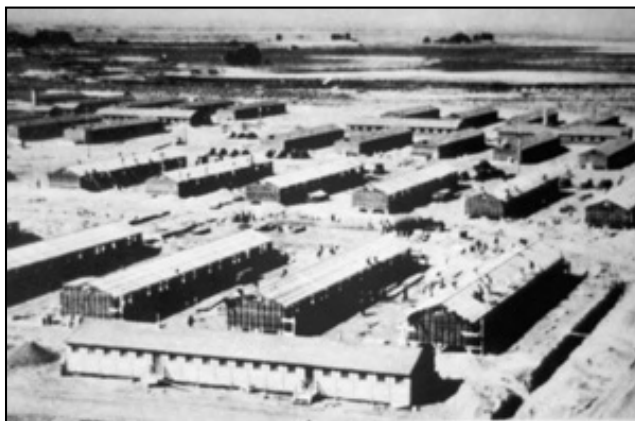
Figure 11.3. Construction underway at the Rohwer Relocation Center.
