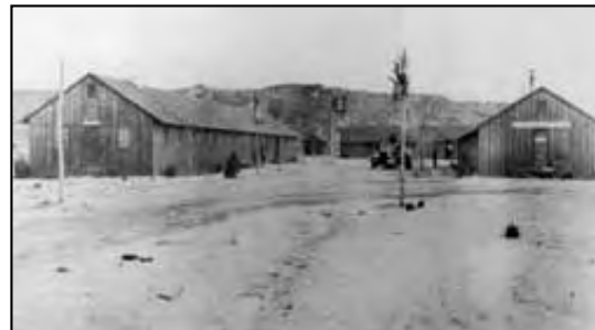
Figure 14.2. Administration building at the Dalton Wells CCC Camp.
