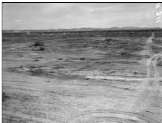
Figure 10.2. Poston site partially cleared. (Clem Albers photograph, Bancroft Library, University of California, Berkeley)
