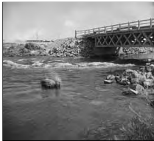
Figure 9.1. North Side Canal.
