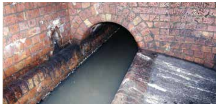
Figure 3.9 – Original Brick Combined Sewer Overflow Chamber
