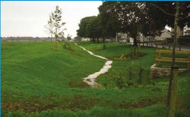
Photos of Swale at Queen Mary's Walk, Llanelli, Wales courtesy of ARUP
