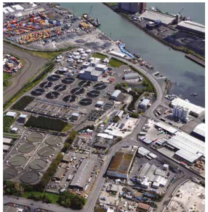
Figure 3.12 - Aerial view of Belfast WwTW
