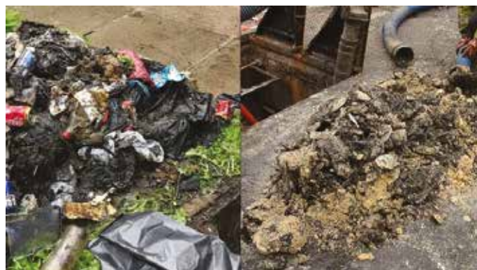
Figure 4.2 - Rubbish items and a fatberg recovered from sewers
