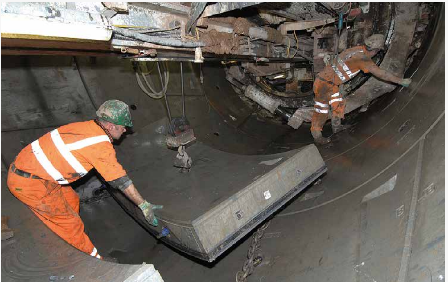
Figure 1: Belfast Storm Tunnel under Construction
