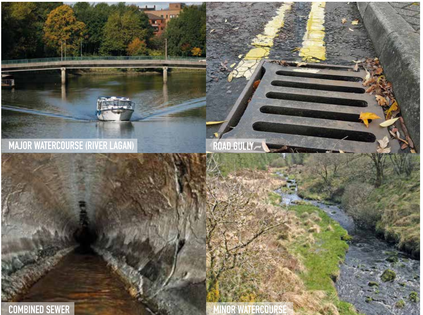
Figure 3.2: Examples of Existing Drainage Infrastructure
