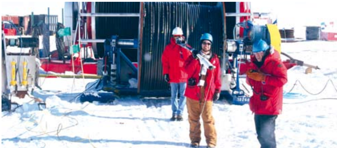
+ Figure 4 Preparing to start deployment of one IceCube string by bringing the end of the Ericsson cable to the drill hole. The large drill hose winch can be seen in the background. Photo: National Science Foundation.
