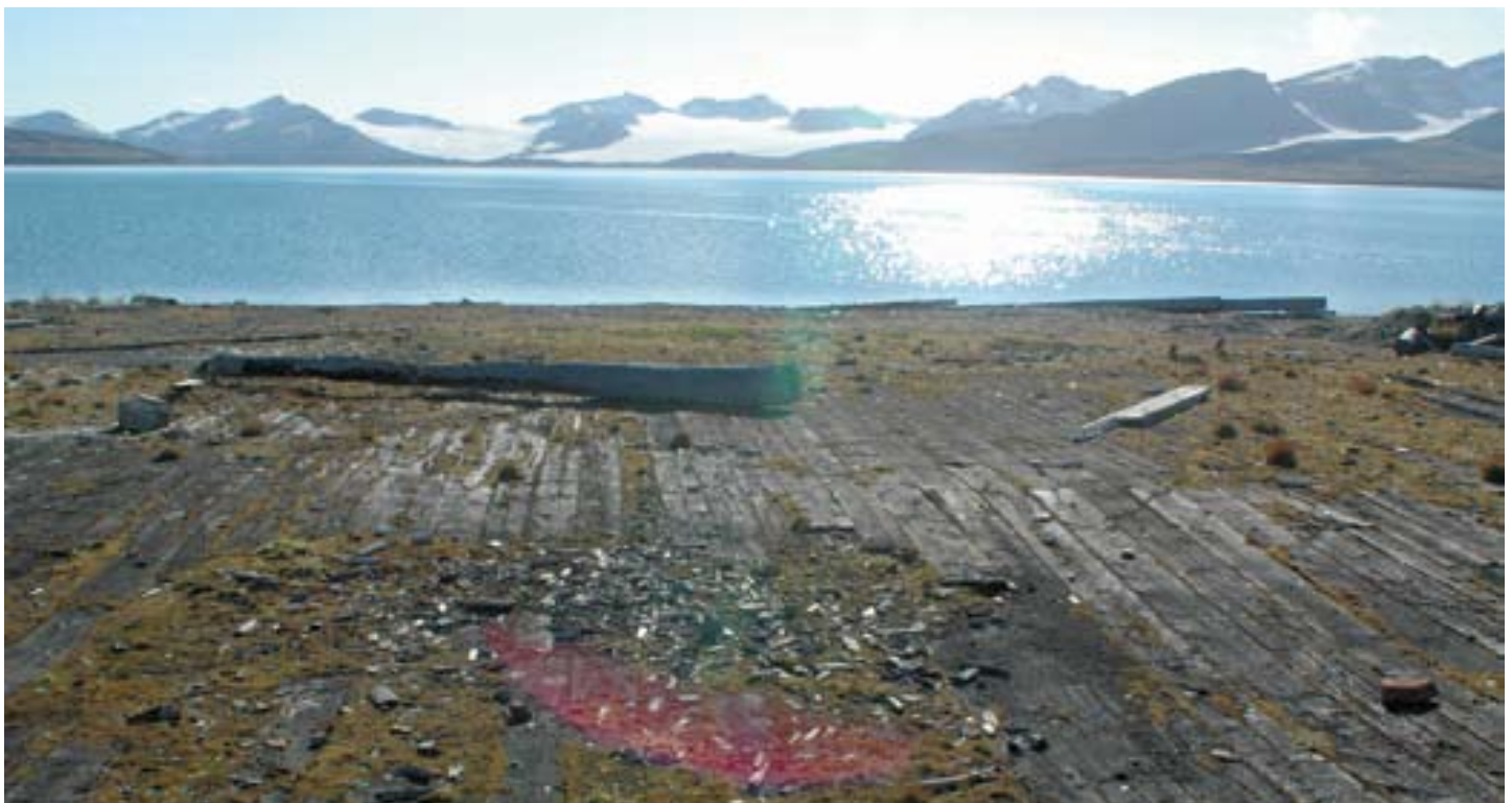
Figure 3 Remains of the flensing plane at Finneset whaling station. The whales were first pulled up on to the floor for cutting, and then further processed in the different production units of the station. Photo: Dag Avango.
