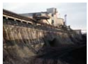
Figure 6 Remains of the concrete foundation for the coal crane of the Nederlandsche Spitsbergen Compagnie from the mid-1920s, re-used today for a conveyer belt by the Russian mining company Trust Arktikugol. Photo: Dag Avango.
